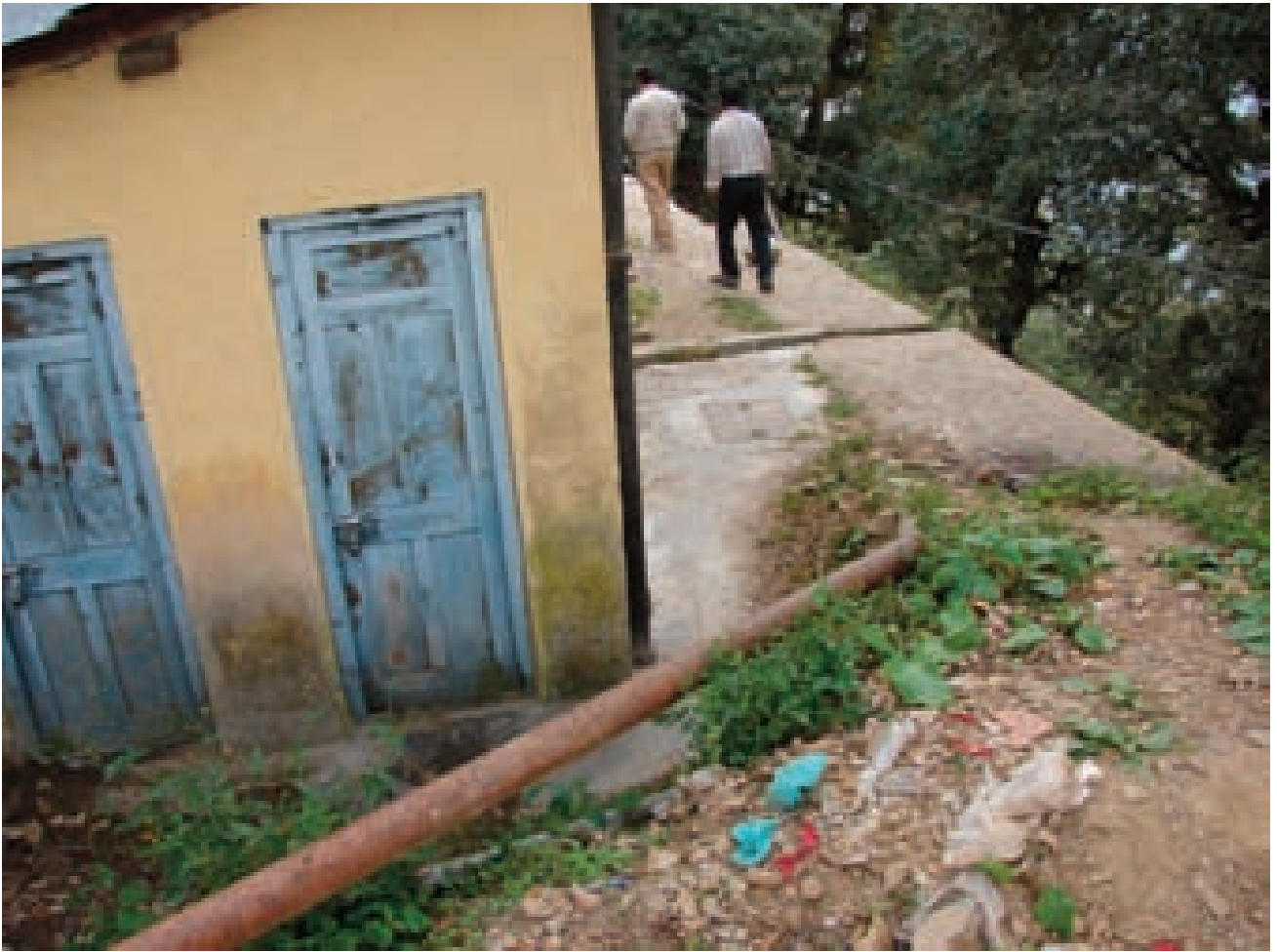
Picture 7 Existing septic tanks at HP state museum
