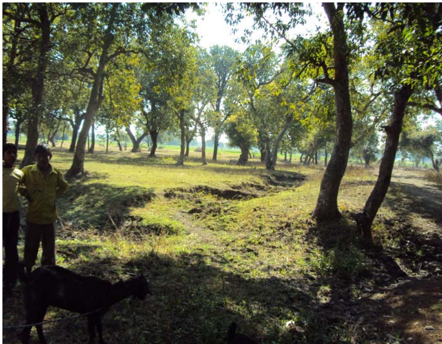
Site selected for Check-dam construction by villagers
