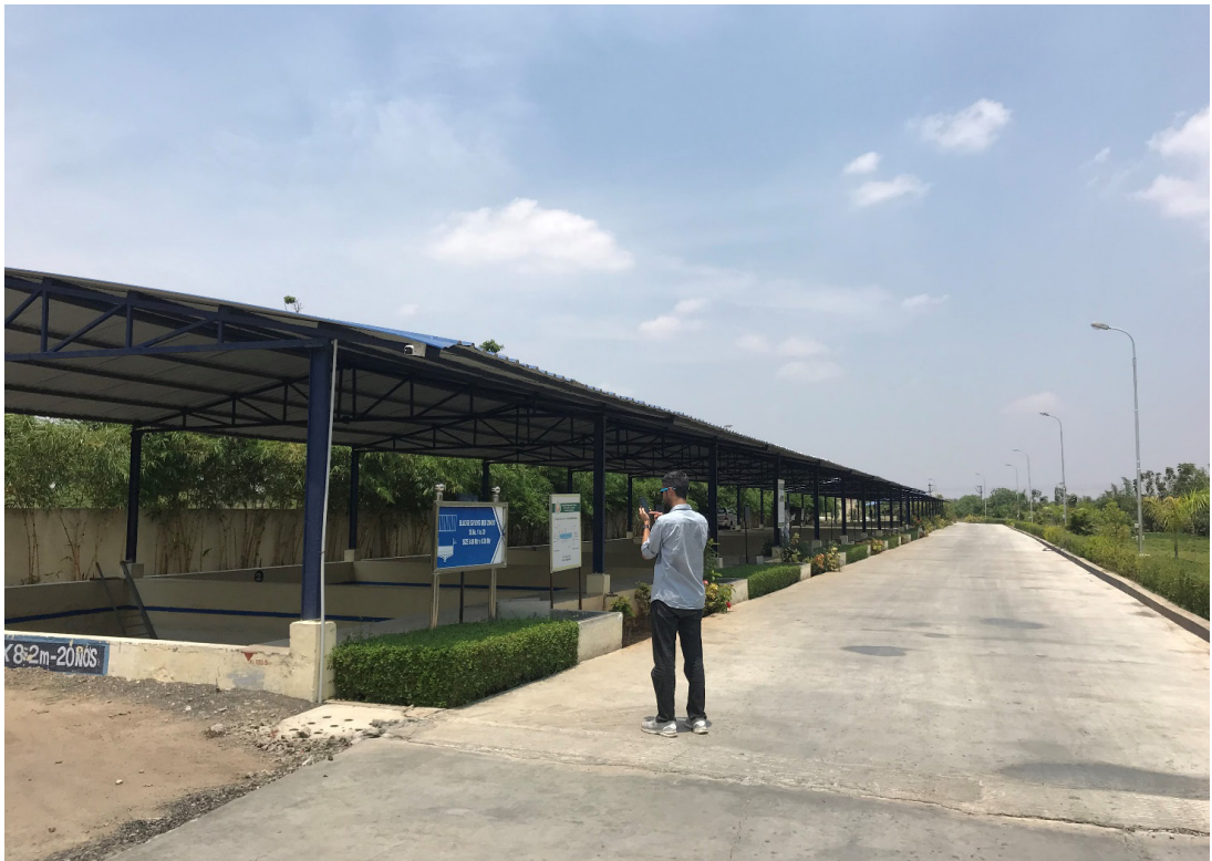
A series of unplanted sludge drying beds at the Karunguzhi FSTP
