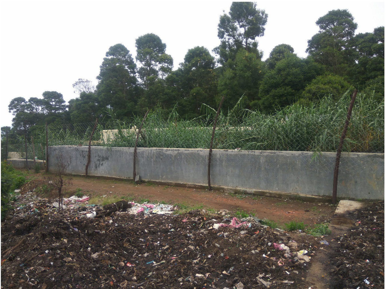
Planted sludge drying bed at the Adigaratty FSTP
