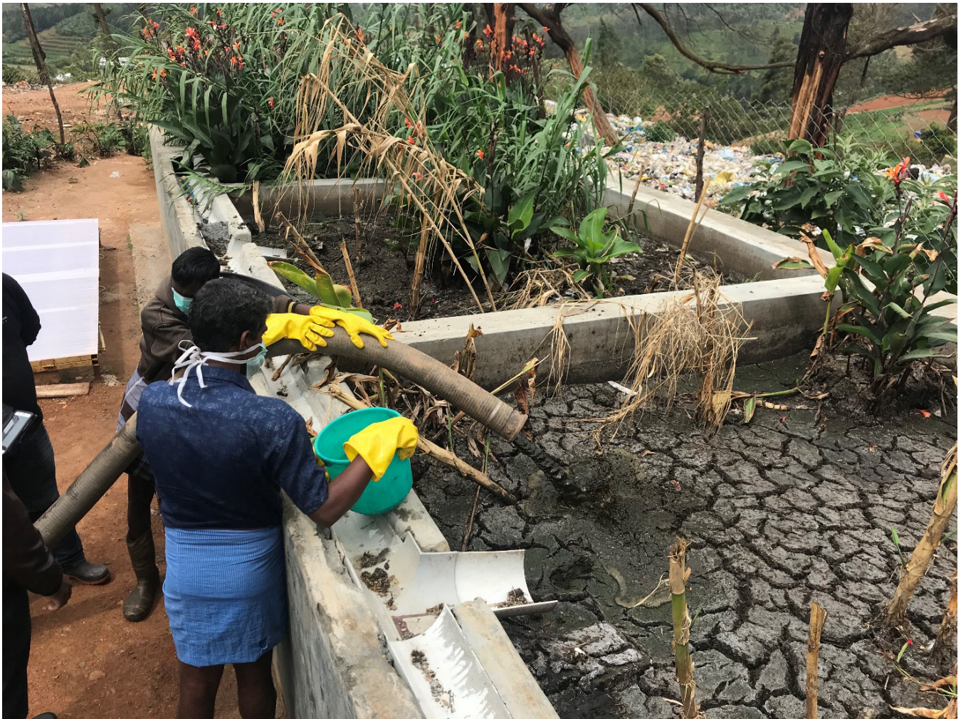
Discharging faecal sludge in the planted sludge drying bed at the Ketty FSTP
