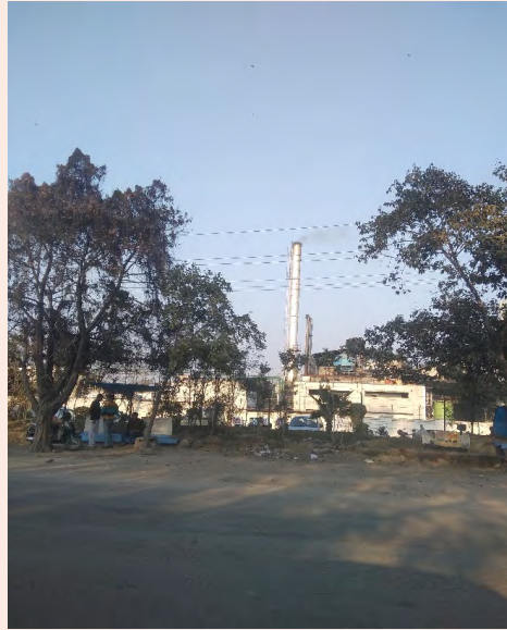
Image 19: Smoke from stack
