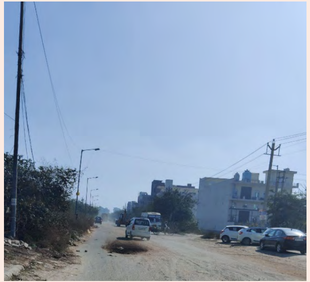
Image 26: Roads in Sonipat Industrial Area
