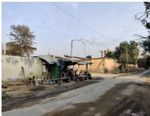
Image 14: Stack emissions and poor road condition in RIICO Industrial Area, Shahjahanpur
