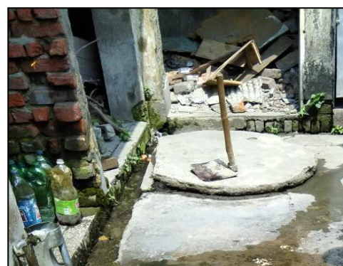
Figure 6: Pit type containment system
