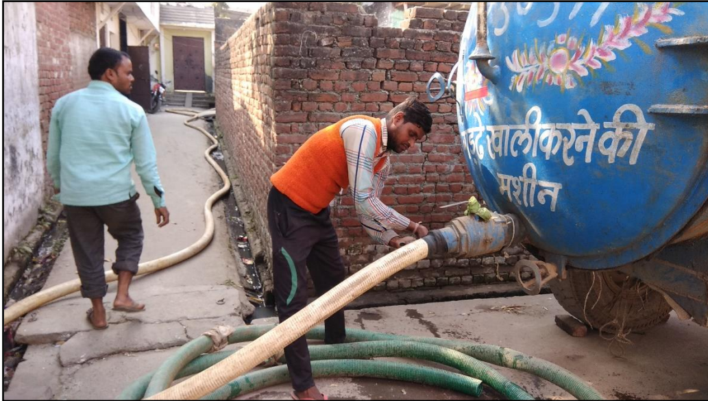
Figure 11: Setting up for an emptying process (Source: CSE, 2017)
