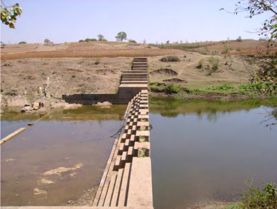
Check dam built across a stream.
