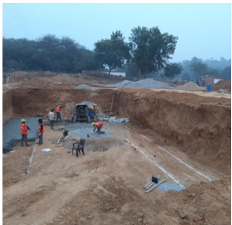
Faecal sludge treatment plant under construction, Chunar
