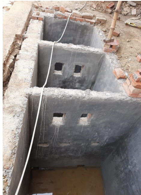
Septic tank under construction, Chunar
