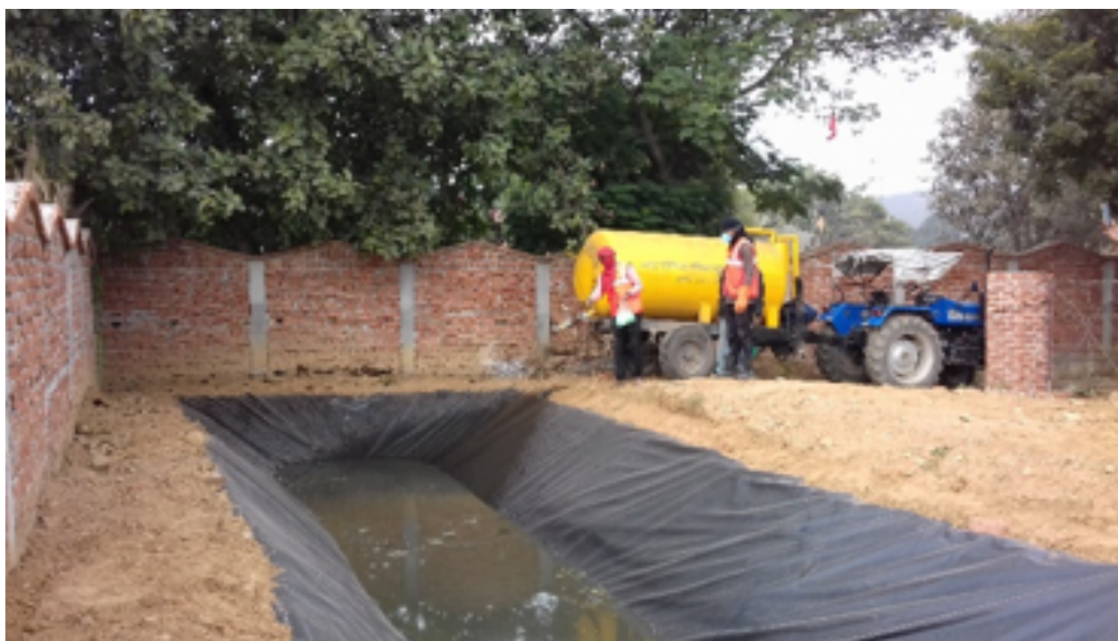
Emptying of faecal sludge at trenching site by government operated vacuum tanker, Chunar
