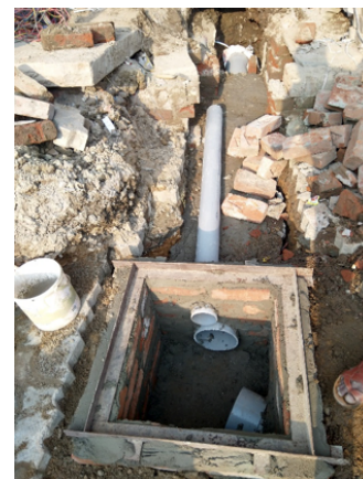
Containment system connected to sewerage network, Prayagraj
