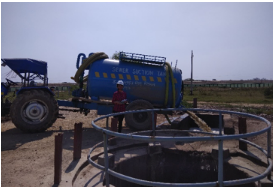
Decanting of faecal sludge at inlet of STP, Kanpur
