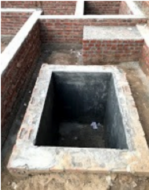
Fully lined tank under construction, Bijnor
