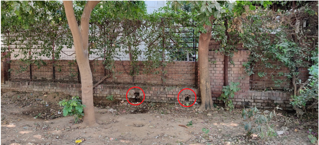
Inflow points for excess run-off from neighbouring Panchsheel Colony
