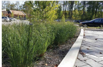
Brookside Gardens: Permeable Pavements
