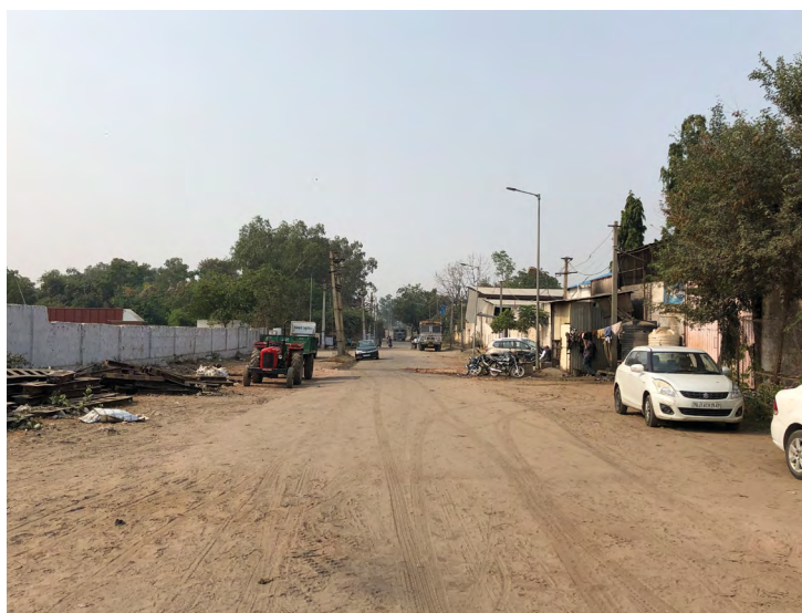
Image 3: Poor road conditions in VKIA.
