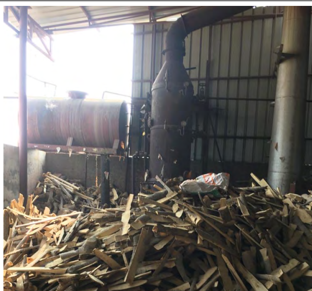
Image 4: Wood waste used as 'fuel' in boilers in Bassi Industrial Area
