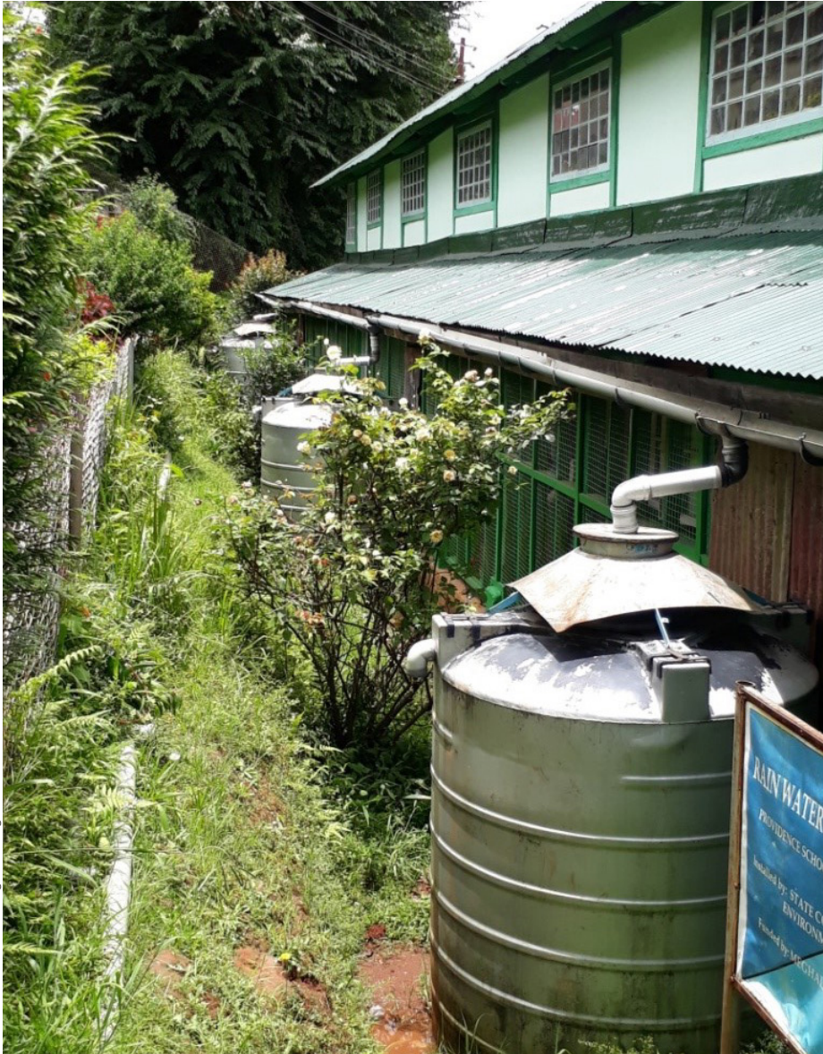
Barrel-type rainwater harvesting system in St. Edmund's College, Shillong collects rainwater from rooftops of buildings
