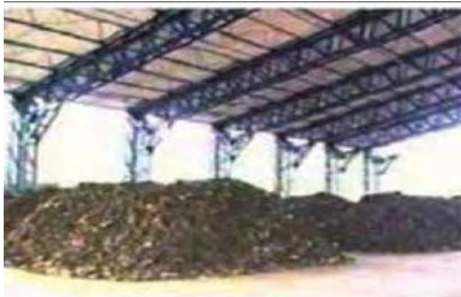
Incoming waste at compost yard
