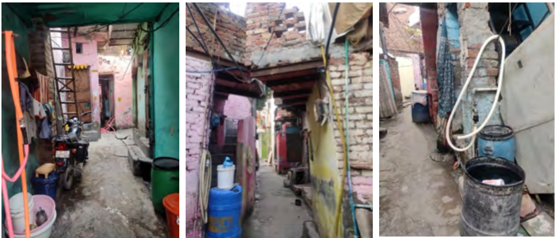
Figure 17: Use of community stand-posts and flexible PVC pipes for access to water supply
