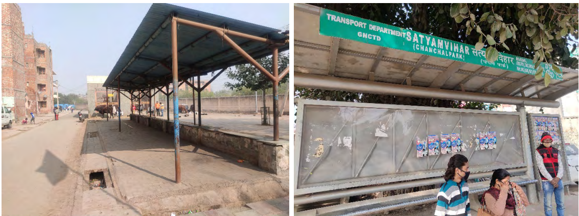
Figure 8: Satyam Vihar (Chanchal Park) bus stop at a distance of about 1 km from Baprola
