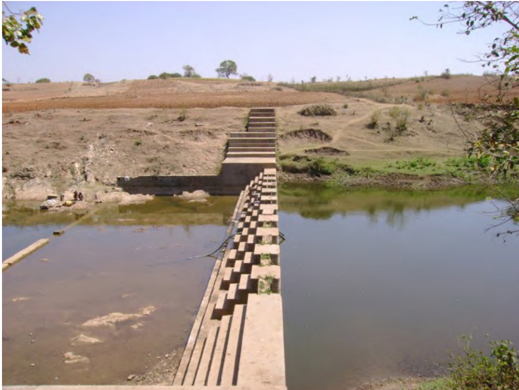
Check dam built across a stream
