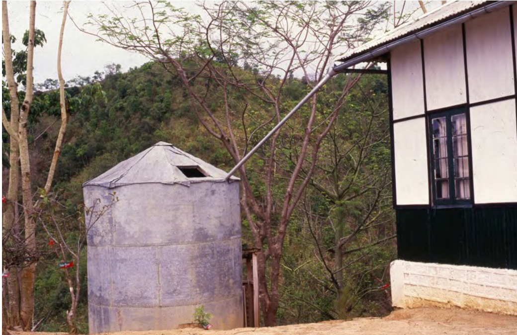
Rooftop rainwater harvesting helps sustain drinking and cooking requirements throughout the year in Northeast India.
