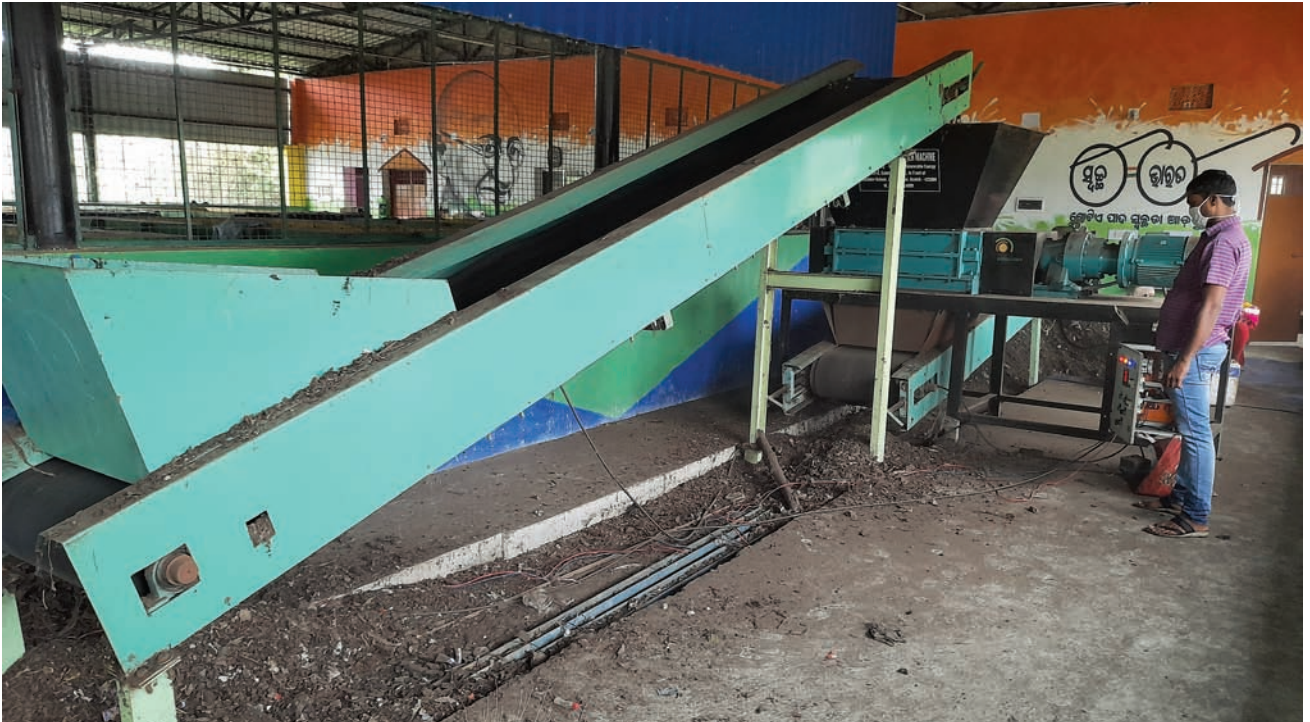
A conveyor belt segregating components of biodegradable waste at a micro-composting centre in Keonjhar
