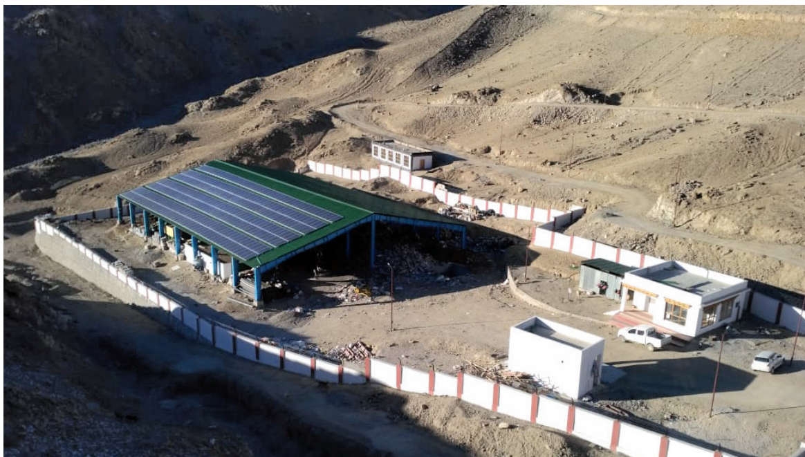
Solar panels installed on the roof of the plant supply sufficient energy for all mechanical operations
