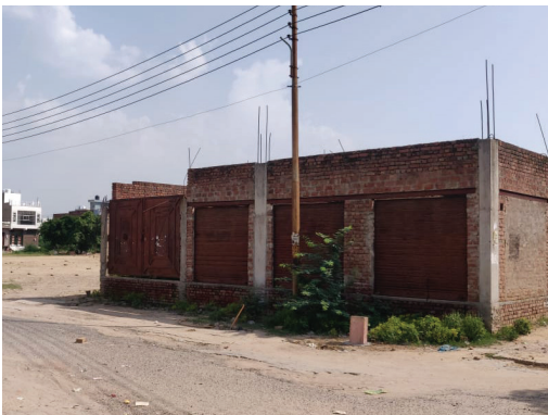
Vacant land allocated for establishment of Petha Nagari in Kalindi Vihar
