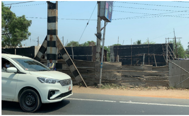
Dust barriers on scaffolding around a building under construction or demolition
