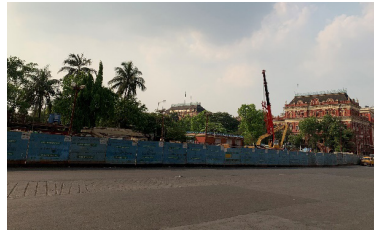
Dust barriers on scaffolding around a building under construction or demolition
