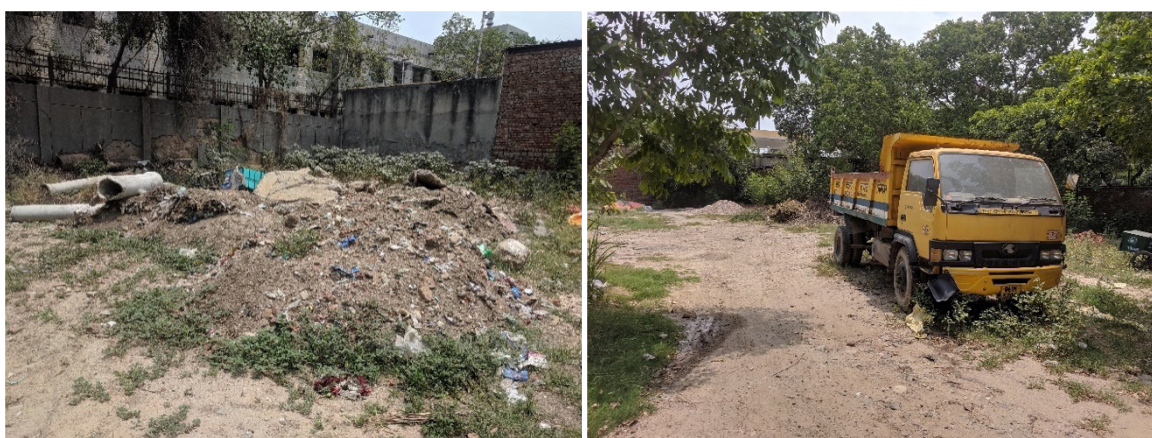
Alipur C&D waste collection point
