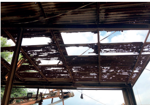
Photographs 16: Partially covered or damaged sheds for dust containment
