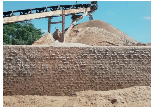
Inadequate height of boundary wall at stone-crushing units
