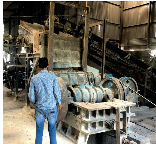
Completely covered sheds for granulators
