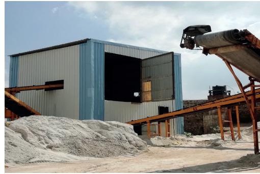
Fully covered shed with doors for maintenance
