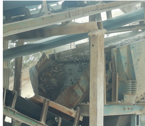
Screening in progress
