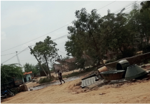
Inadequate boundary wall height
