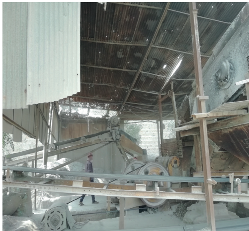
Partially covered sheds
