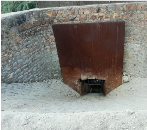
Unloading point for raw material (deep pit feeder)
