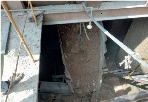
Photograph 17: Non-operational sprinklers
