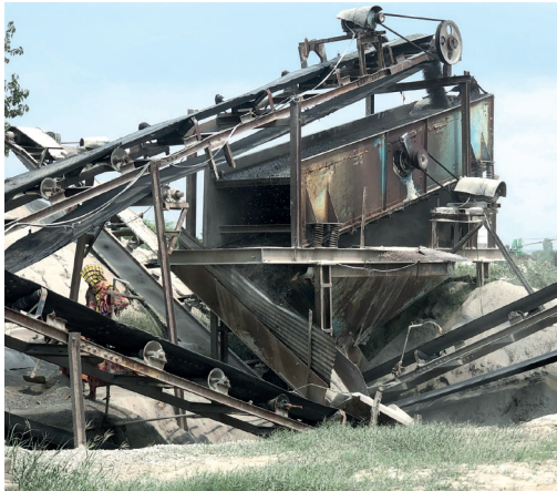
Typical screening unit
