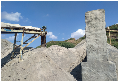
Conveyor belt covered with thick cloth
