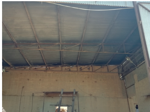
Fully covered shed with door
