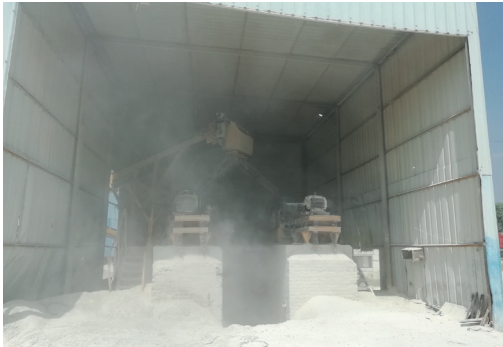
Photograph 14: Fugitive dust from tertiary process
