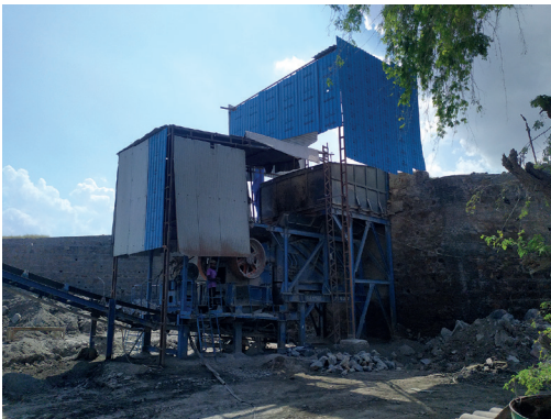
Partially covered shed
