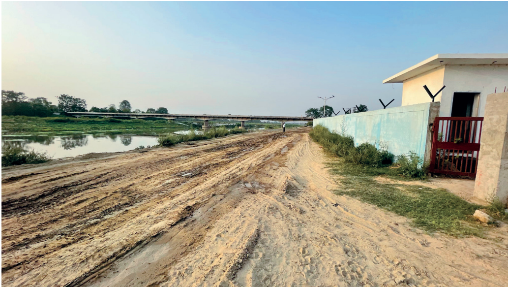
An FSTP site located close to a river (flood-prone area).
