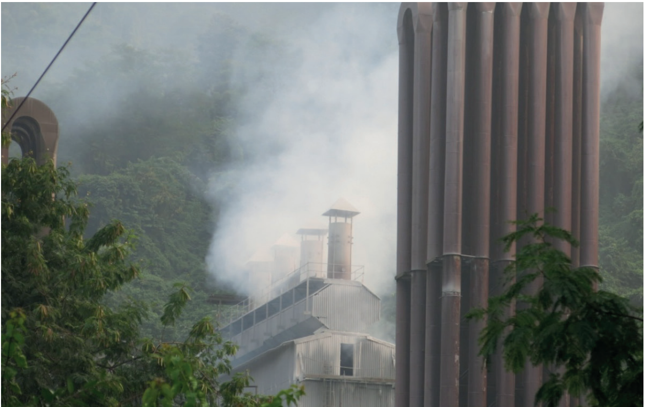
Figure 33: Emission from point source during non-operation of Gas Cleaning Plant
