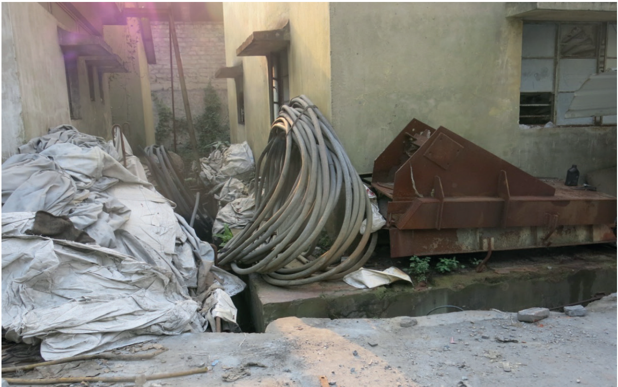
Figure 23: Poor housekeeping – storage of waste without any designated place
