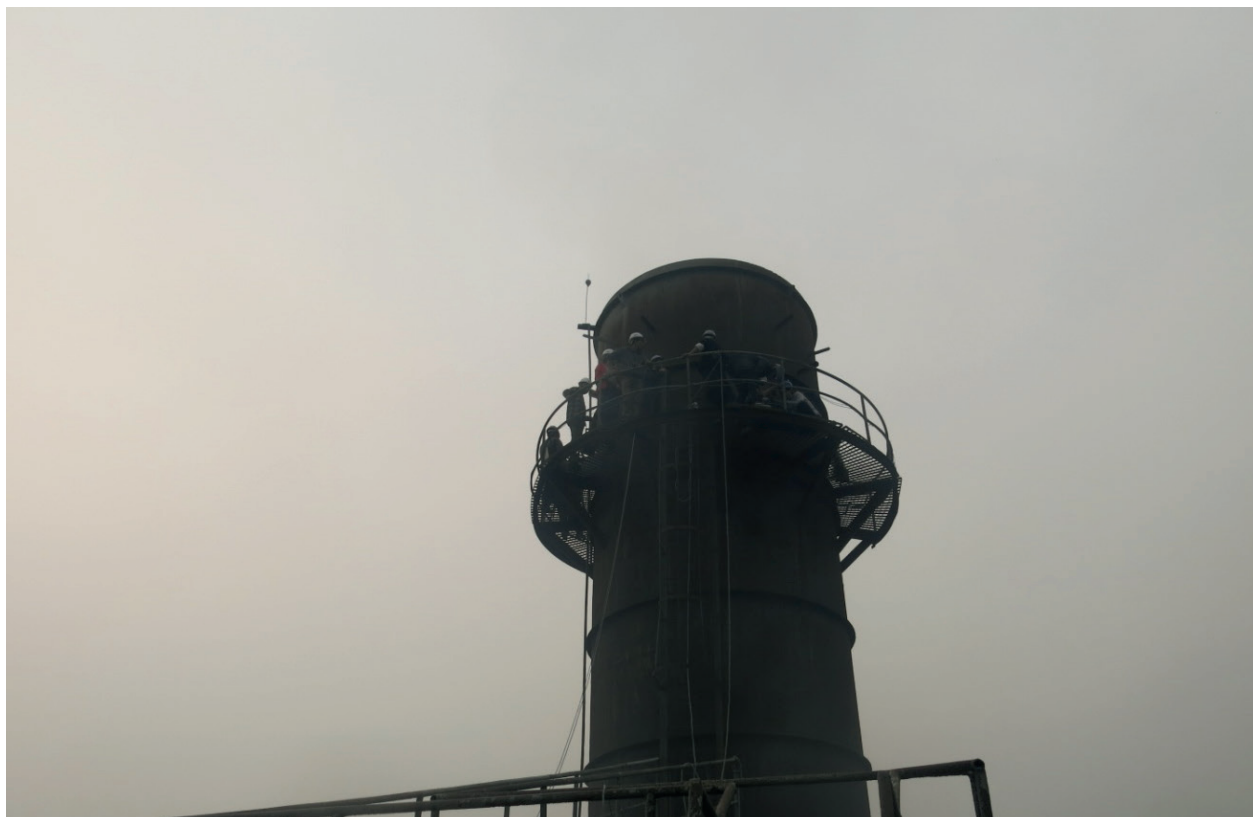
Figure 6: Monitoring of point source emission at a stack
