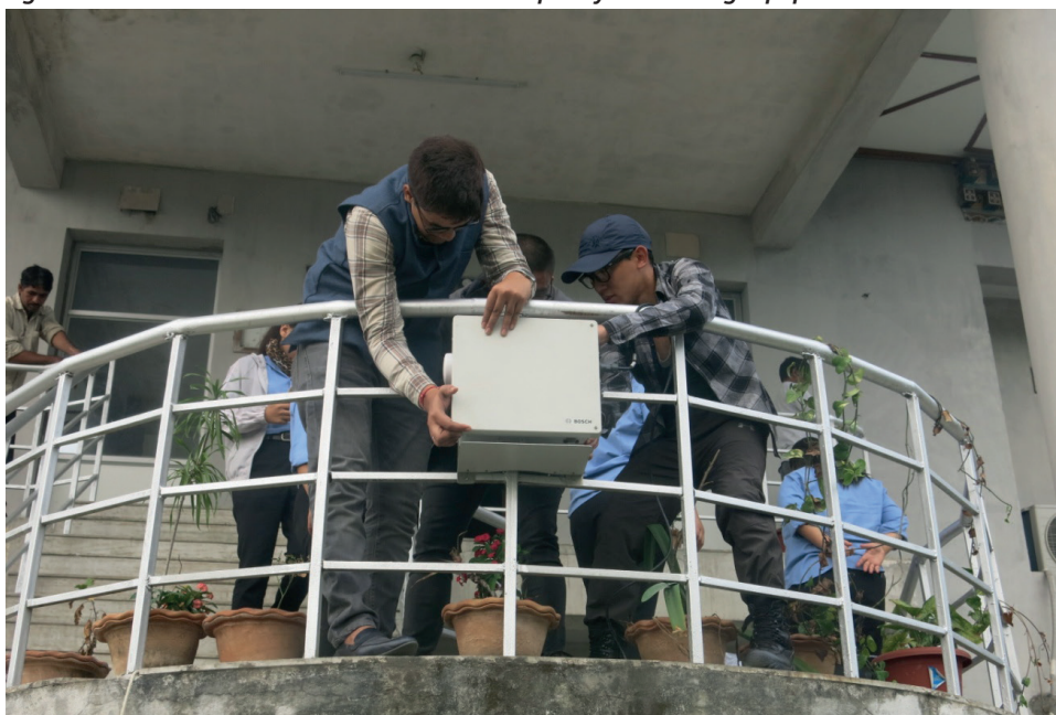
Figure 5: Installation of continuous ambient air quality monitoring equipment near IIDD office
