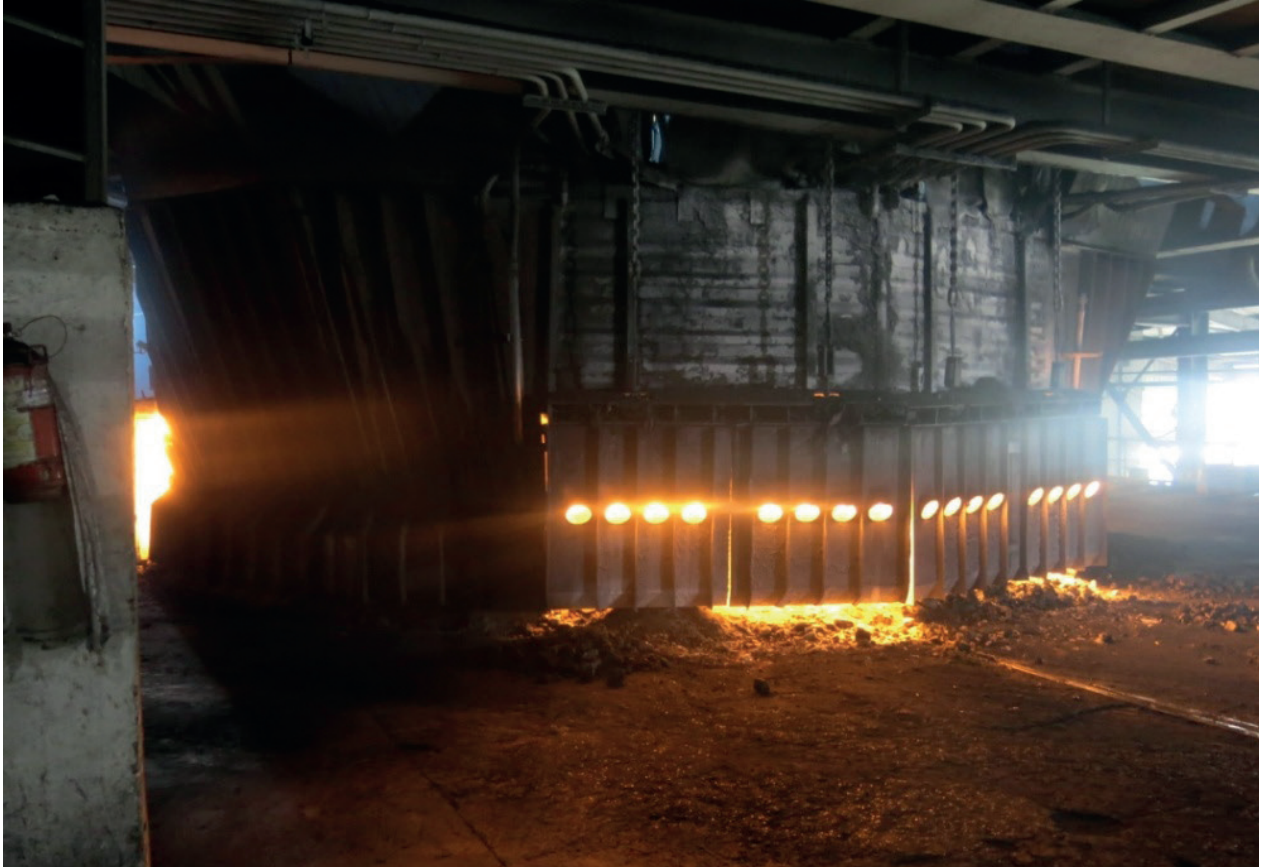
Figure 16: Hydraulically operated furnace doors at a submerged arc furnace—Reduces fugitive emission
