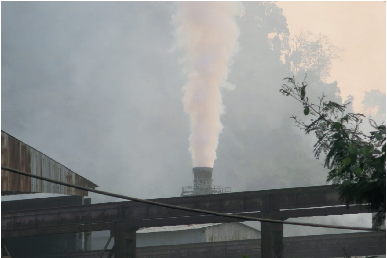
Figure 34: Emission from point source during non-operation of Gas Cleaning Plant
