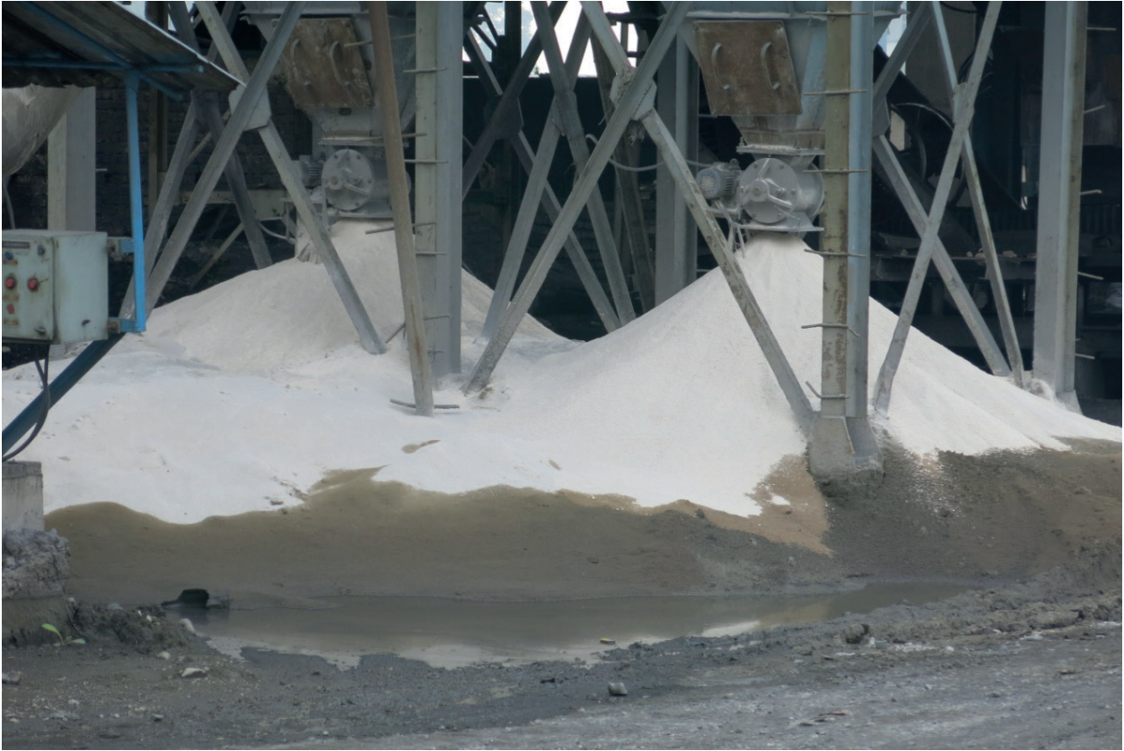
Figure 32: Poor dust handling mechanism from hoppers of gas cleaning plants
