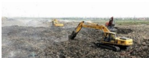
Figure 7: Steps involved in dumpsite remediation
