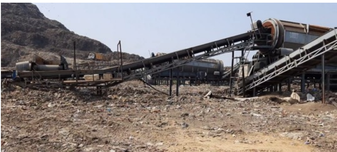
Conveyors at a legacy waste treatment site
