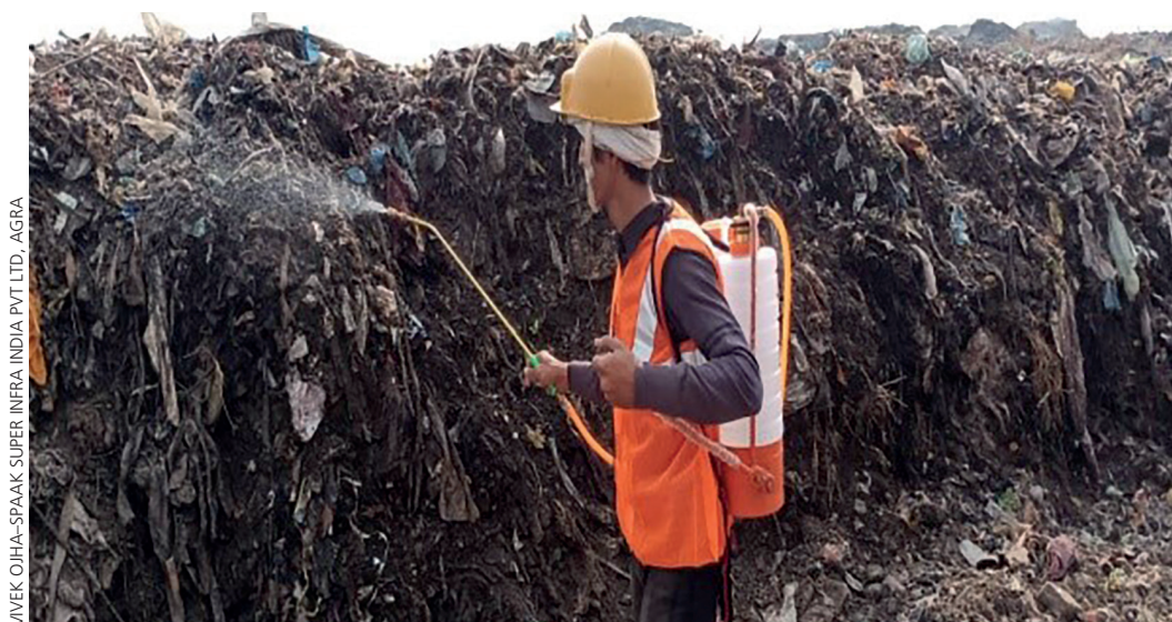
Spraying of bio-inoculum during stabilization of legacy waste
