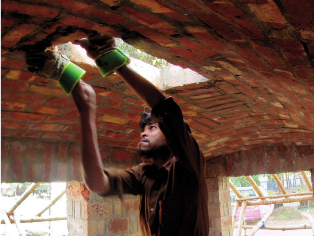
A mason constructing a shallow dome using bricks
