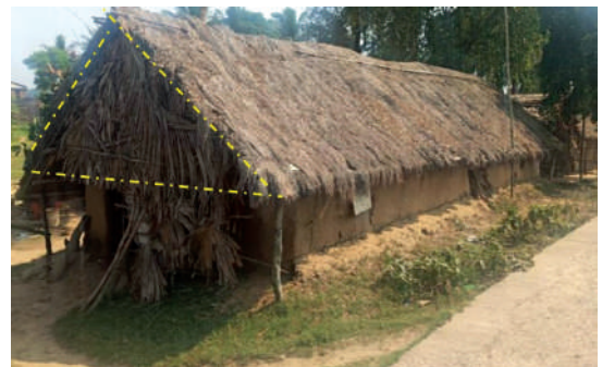
Dwellings with pitched roofs that have increased slopes and longer sides which are aligned with the direction of the wind.
