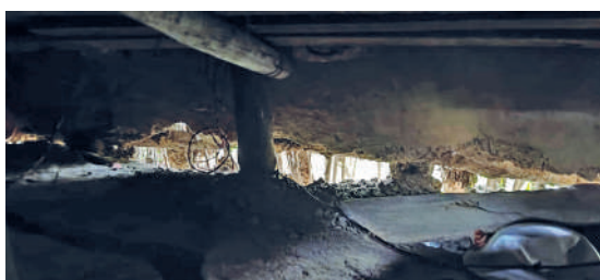
The base of wattle and daub walls cracked open due to the frequent floods in Purba Sridharpur
