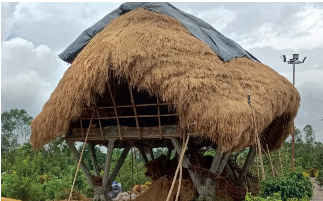
Roof made from bamboo and rice thatch in Purba Sridharpur, Sunderbans
