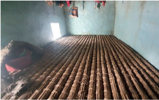
Flooring members made out of bundles of sor grass in Bolpur
