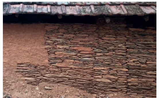
Slat stone coursework:
