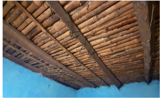
Bamboo and wood used for intermediate flooring in Bolpur
