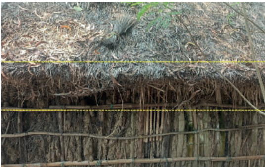
Thatched roof with fishing nets layered over it
