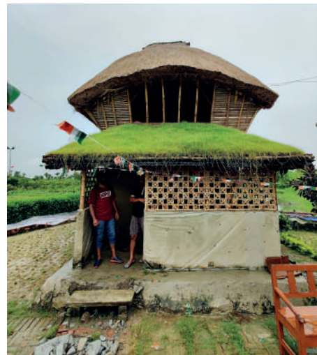
House prototype 3 uses wattle-and-daub construction and thatch for the roof
