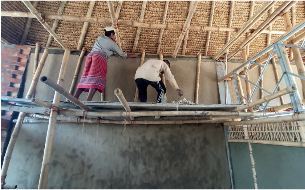
Wall construction in Free Residential School, Joka, Kolkata
