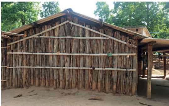
In Balliguda, Odisha, wood panel walls are used with mud plaster
