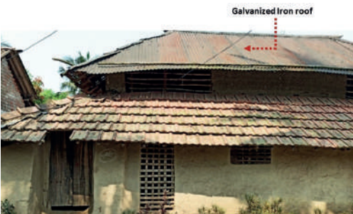
Transition technologies—galvanized iron roof
