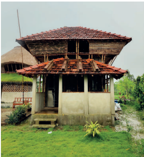
House prototype 2 uses Hydraform blocks and flat terracotta tiles
