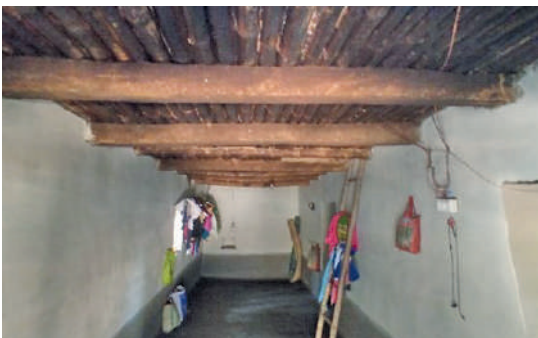
Wooden beams crossing the span of the room with bamboo laid on top
