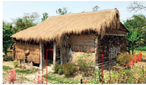
Brick walls with thatch roof in Purb Sridharpur
