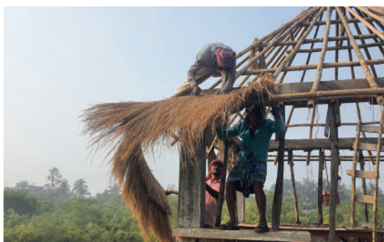
Masons putting up thatch panels for roofing
