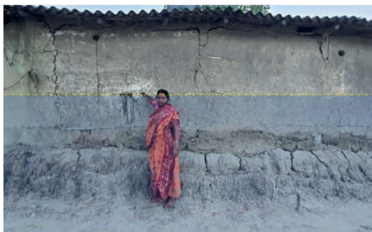
The height of flood waters and impact of flooding on houses near Purba Sridharpur
