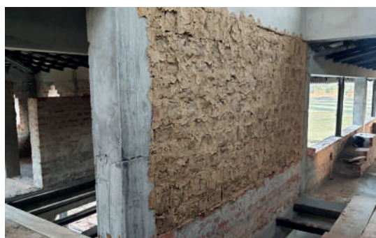
Adobe brick infill wall in portal structures
