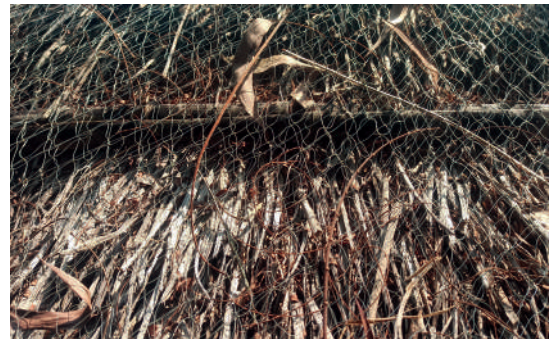
Fishing nets tied over roof structures
