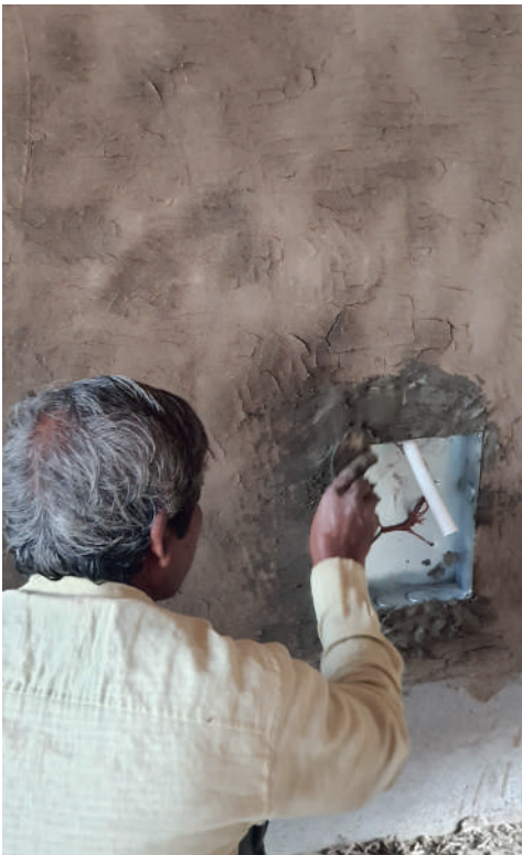
Modern electric services being inserted in bamboo wall construction
