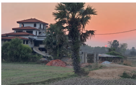
Unnamed house by Bidyut Roy, Bolpur, West Bengal
