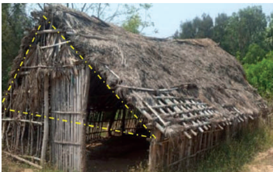
Dwellings with pitched roofs that have increased slopes and longer sides which are aligned with the direction of the wind.
