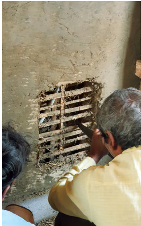
Modern electric services being inserted in bamboo wall construction
