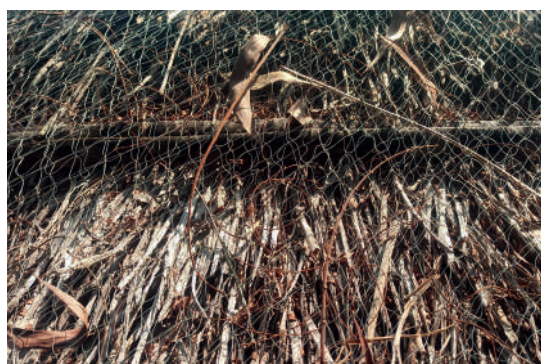
Fishing nets are used over roof thatches to provide resistance to wind in Gundalba, Puri
