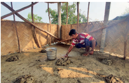
Mason making a mud-cow dung floor
