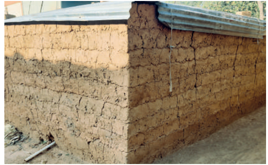
Layered mud walls in Bolpur
