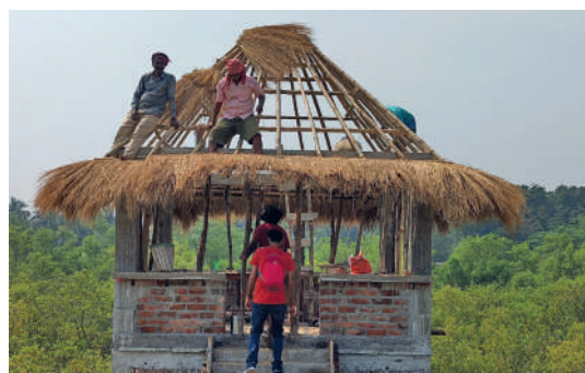
Masons putting up thatch panels for roofing
