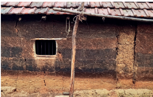
Mud brick coursework and laterite columns in Baripada, highlands of Simlipal
