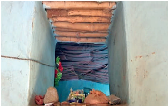
Bamboo lintel in cob-wall construction
