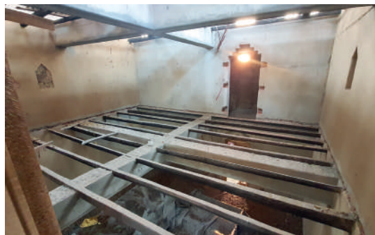
Wood and concrete structural framework
