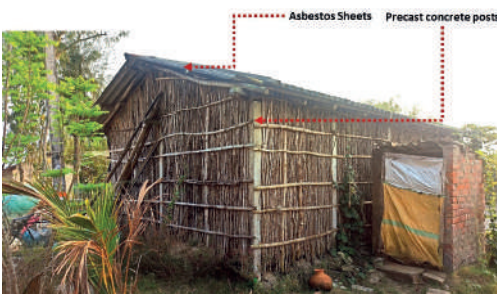
A hybrid of concrete pillars with wattle-and-daub walls
