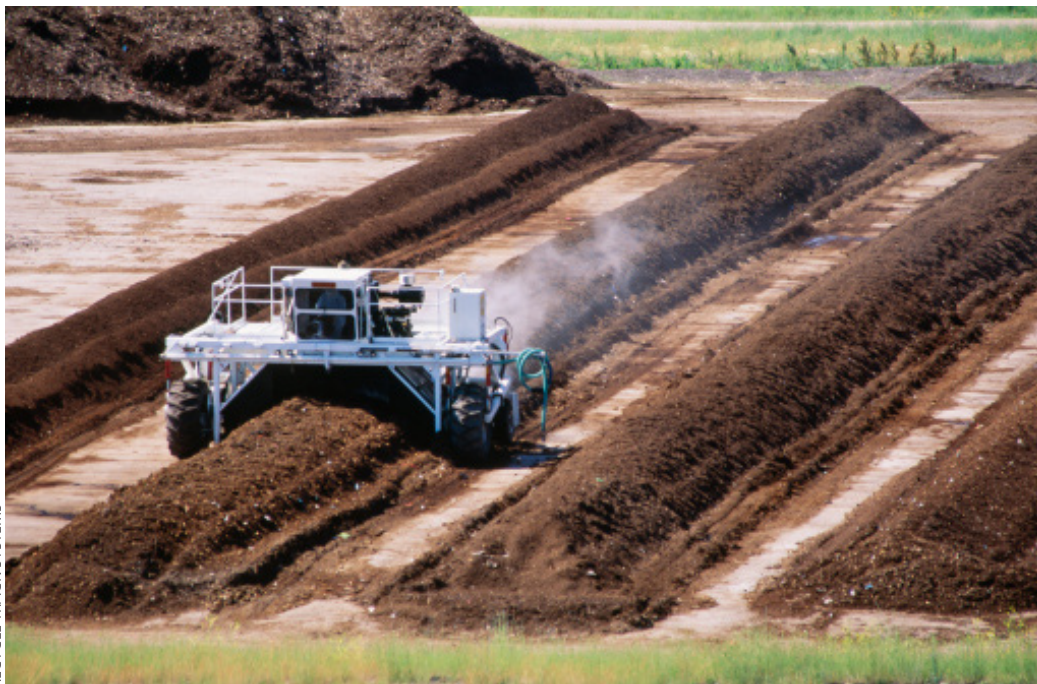
Industrial composting facility
