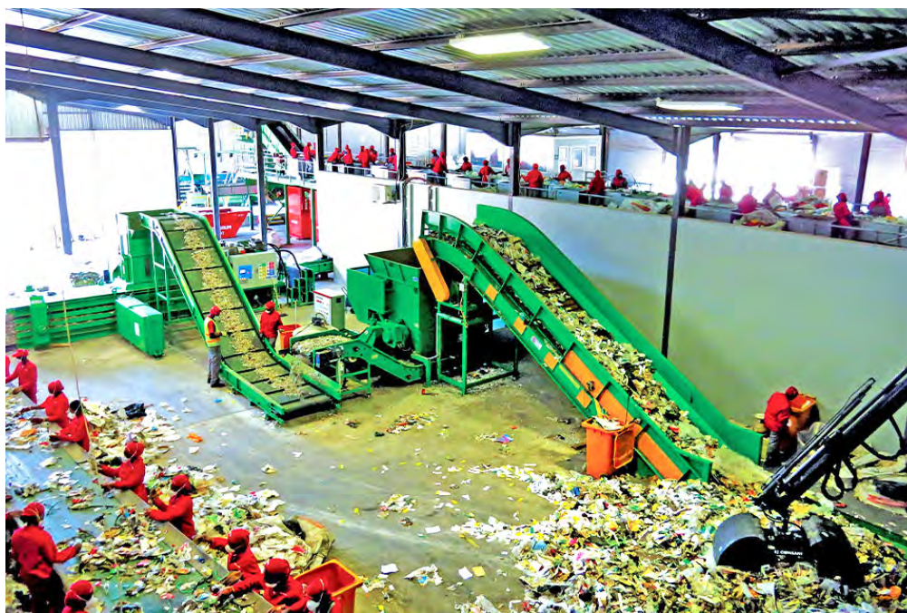
Material recovery facility owned and operated by Rent-a-Drum in Windhoek city
