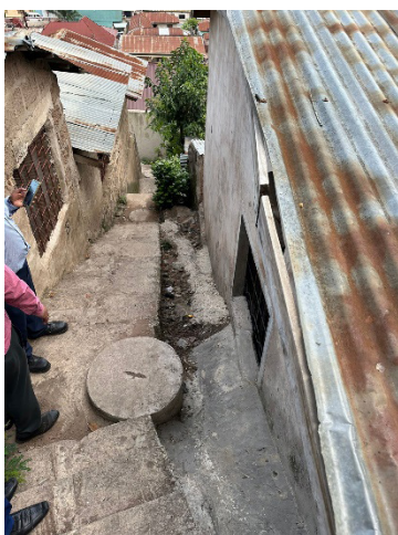
Simplified sewers connected to households on the hills
