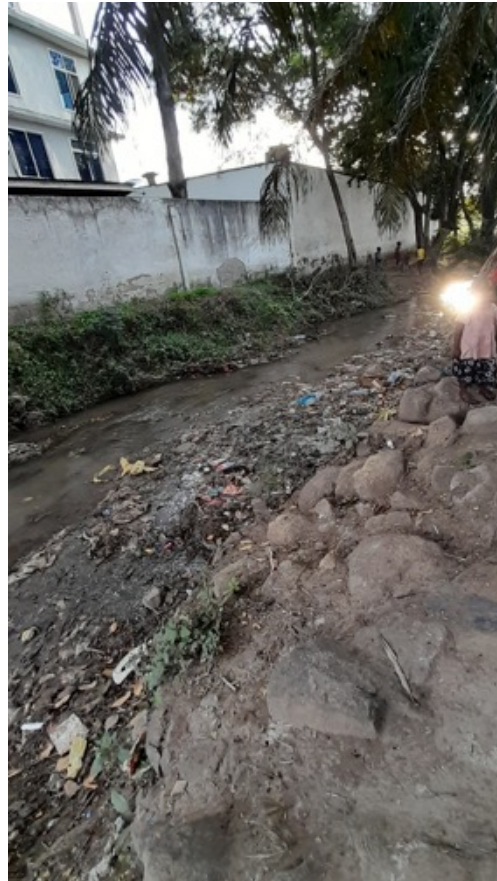
Waste dumped at Mkuyuni drain
