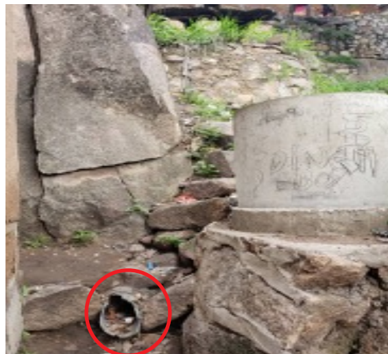
Hidden outlets of lined tanks with impermeable walls and an open bottom
