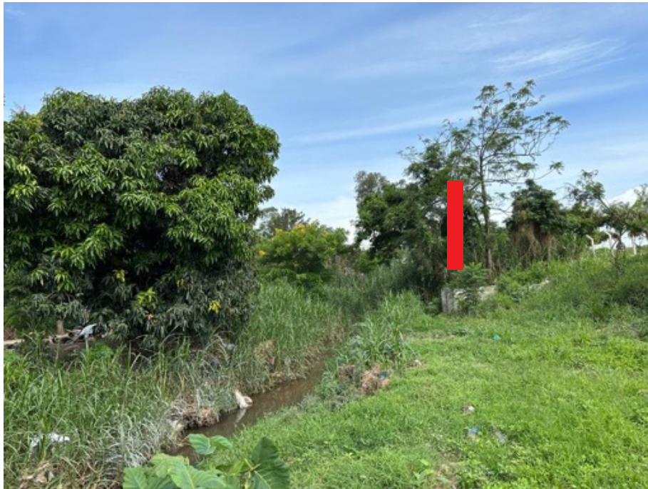
Discharge of effluent from a waste stabilization pond to a stream
