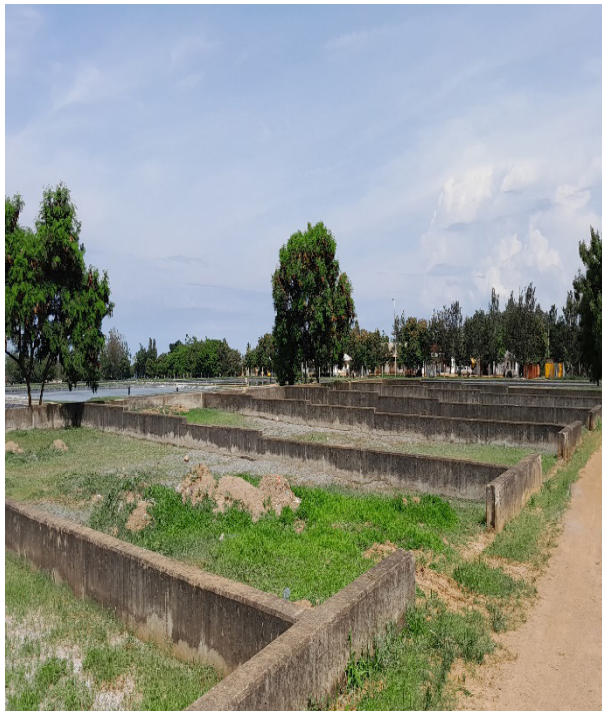
Defunct sludge drying beds
