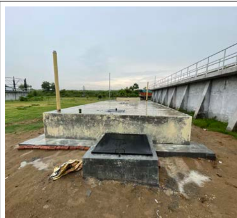
Photograph 17: Completed control valve chamber with cover
