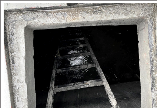
Photograph 9: Ladder Installed in HT chamber
