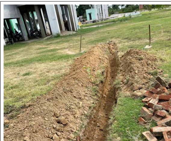
Photograph 12: Excavation of trench for laying leachate pipe
