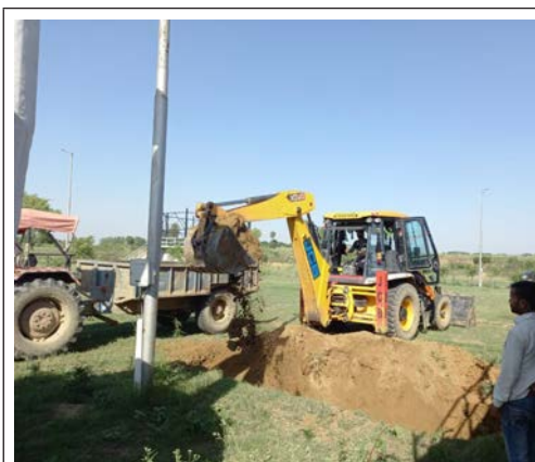
Photograph 6: Excavation for the homogenization tank
