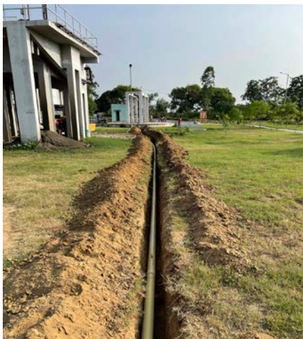
Photograph 14: Pipe laid in the trench
