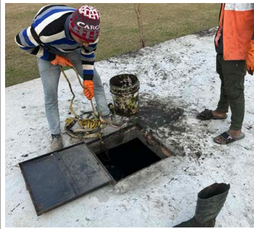
Photograph 2: Removal of accumulated sludge
