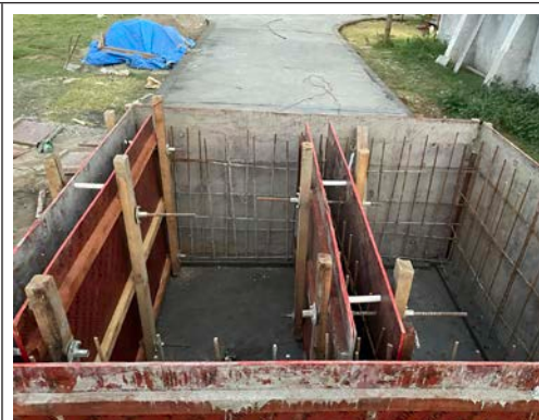
Photograph 11: Rectified setting of the SC
