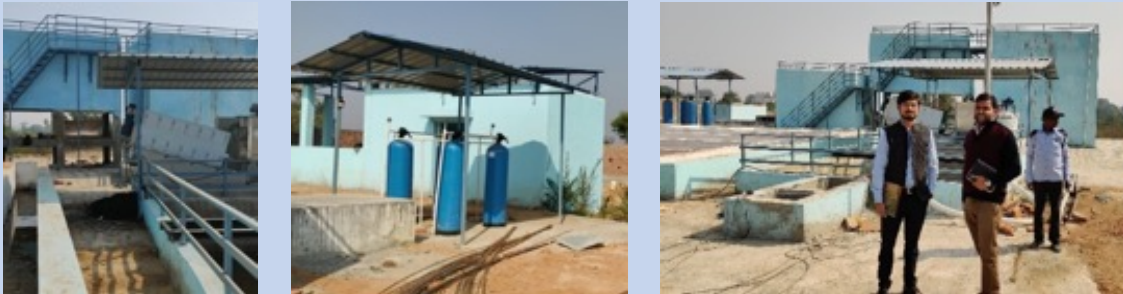
Photograph 10: Photos of 32 KLD FSTP
