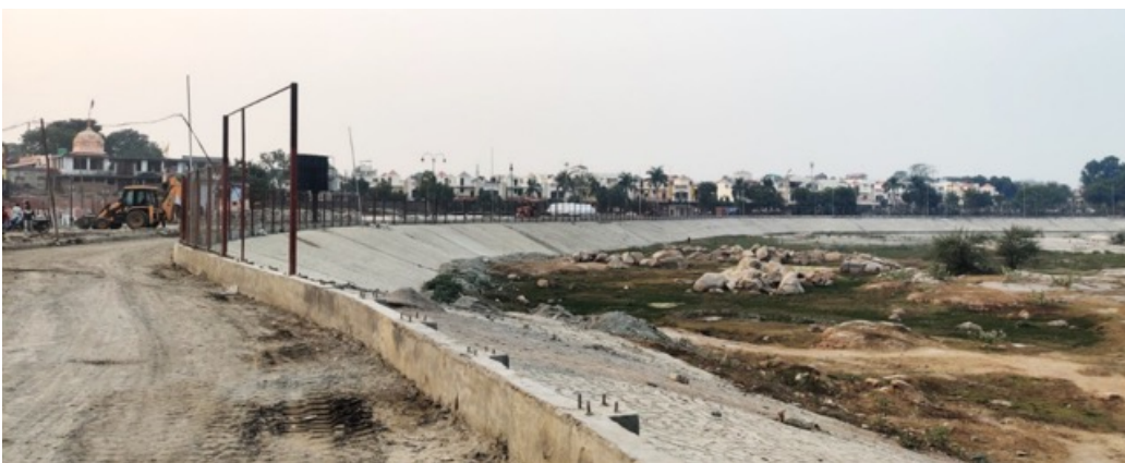
Photograph 26: Restoration work in progress
