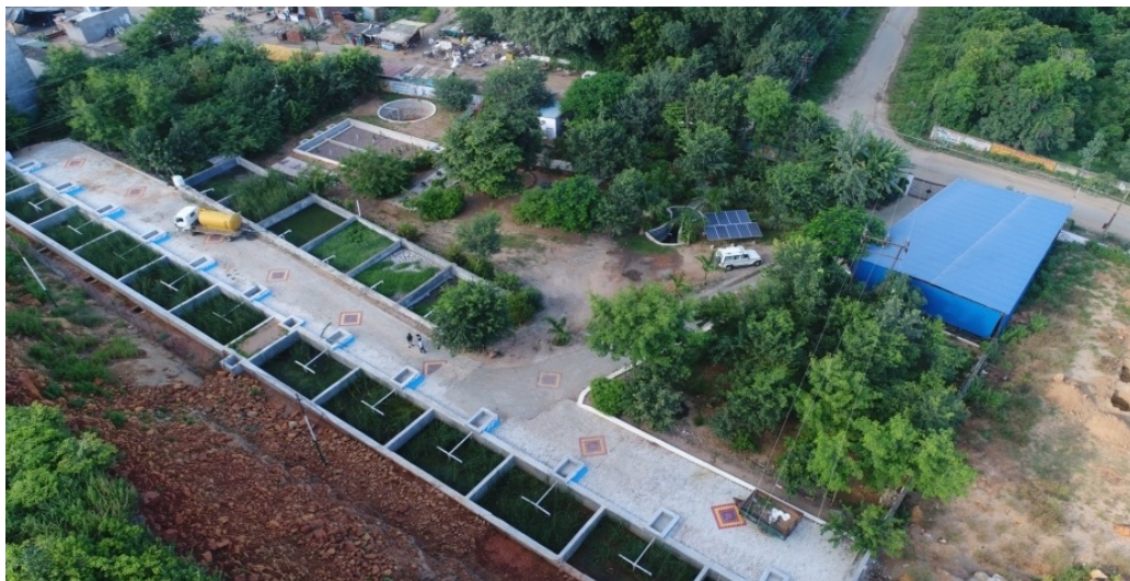
Photograph 5: Faecal Sludge Treatment Plant (6+12 KLD), Jhansi
