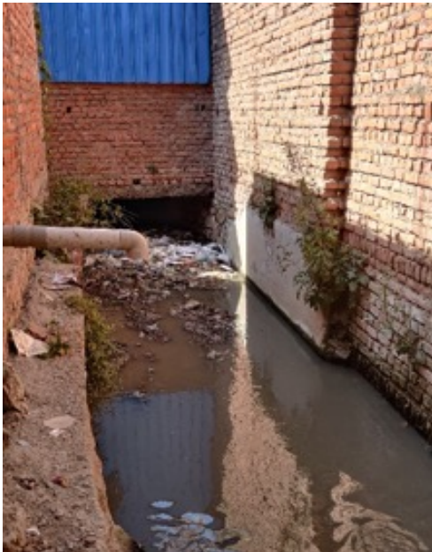
Photograph 30: Encroachment and direct discharge of wastewater into a drain in Shivaji Nagar
