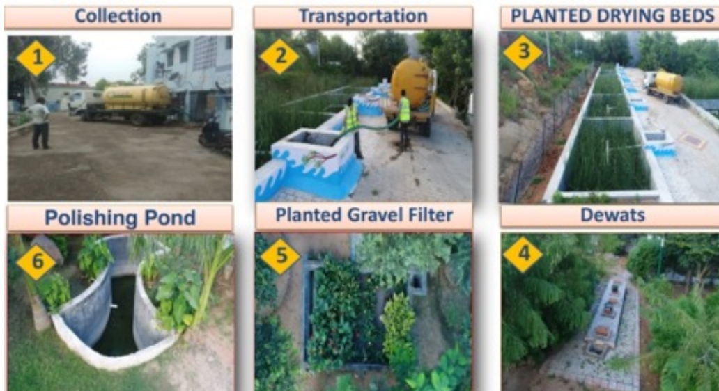
Photograph 4: Faecal sludge and septage treatment process in Jhansi
