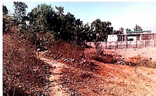
Photograph 2: FSTP Site (6+12KLD)
