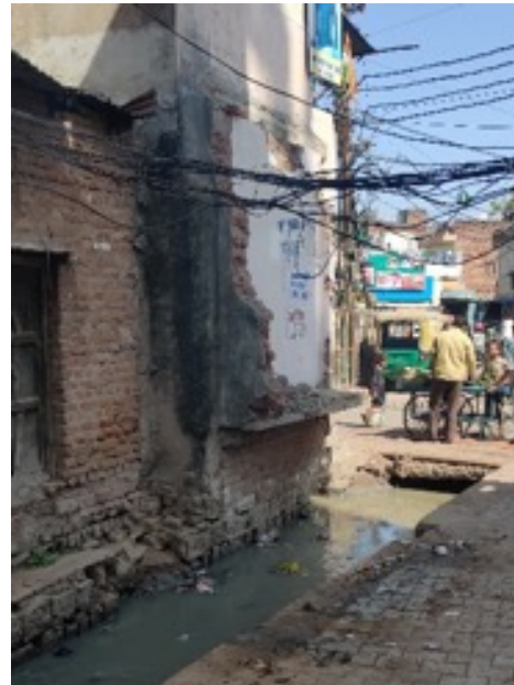
Photograph 31: Removal of encroachment over Kasai Mandi Nallah
