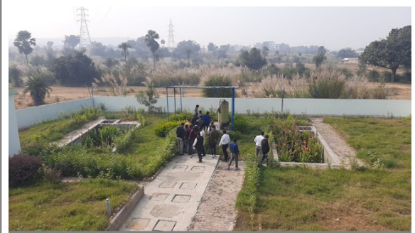
Photograph 20: Liquid treatment unit
