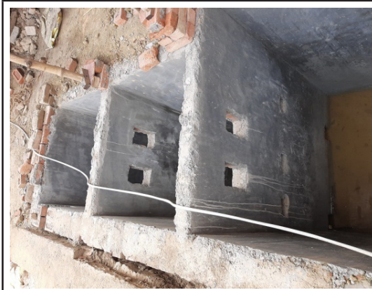
Photograph 1: Septic tank under construction in Chunar
