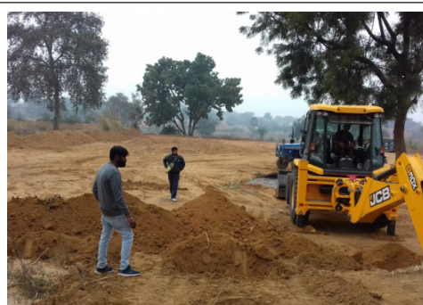
Photograph 6: Excavation at the FSSTP site
