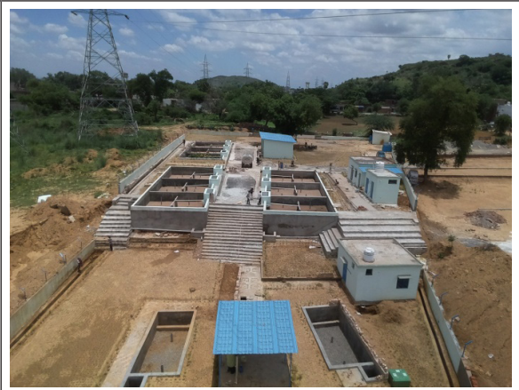
Photograph 18: Construction of the FSSTP in Chunar in progress
