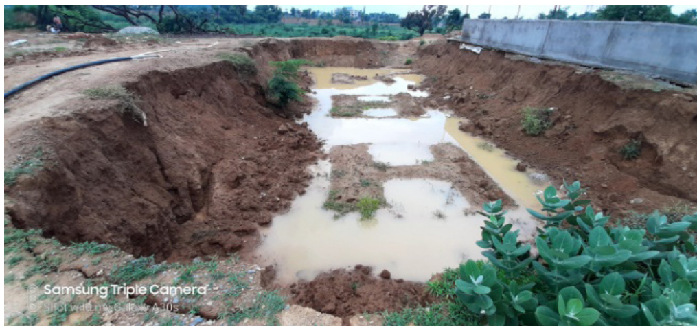
Photograph 9: Construction of planted drying beds hampered by rain
