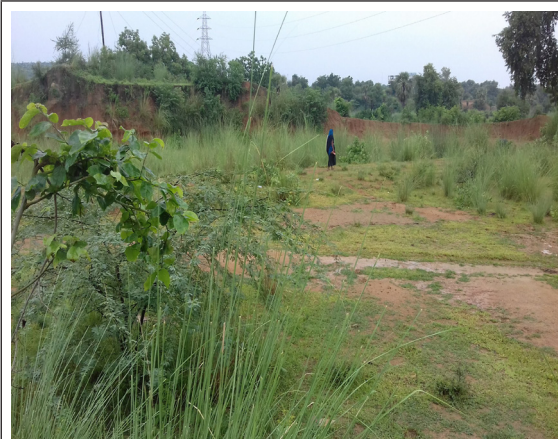
Photograph 17: Before construction of the faecal sludge and septage treatment plant (FSSTP)
