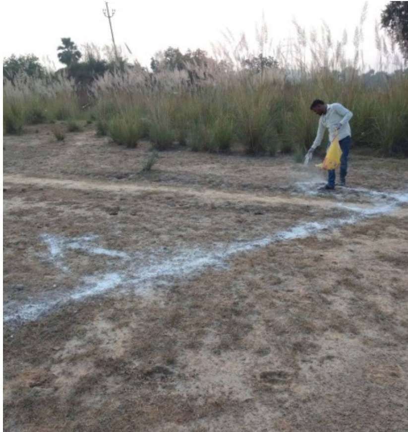
Photograph 4: Demarcation of the site for the proposed faecal sludge and septage treatment plant (FSSTP)
