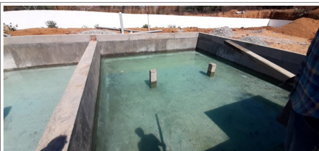
Photograph 13: Hydraulic tests were carried out to ensure the structure was leak-proof
