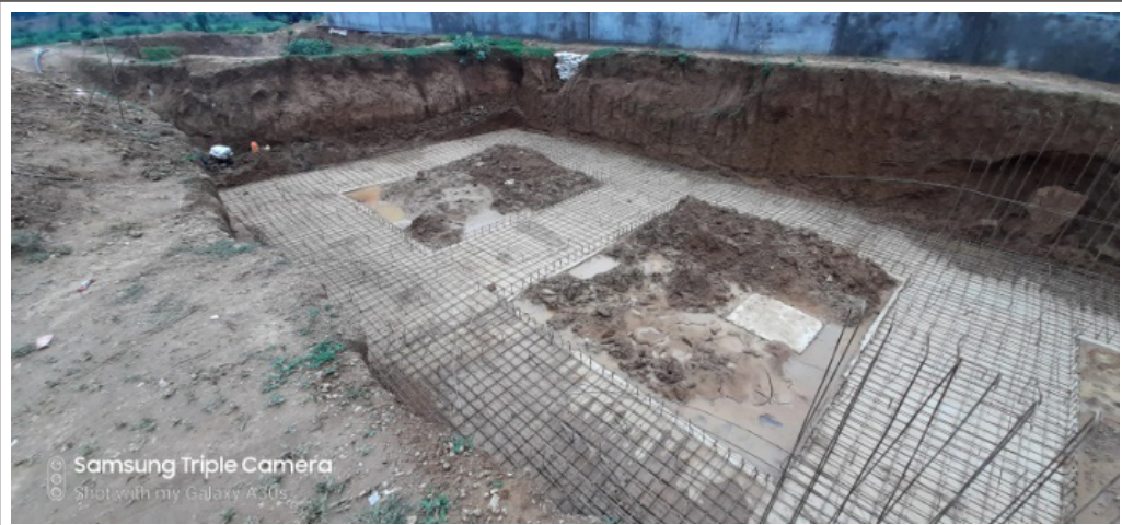
Photograph 8: Construction of planted drying beds (PDBs)
