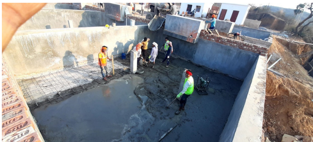
Photograph 10: Laying concrete in planted drying beds
