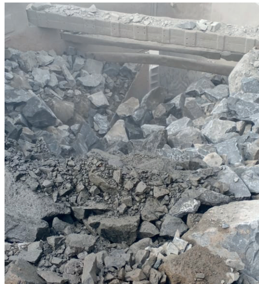
3b. Unloading of material through trucks in feeders
