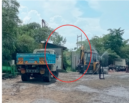
9b. Wind-breaking wall of inadequate height
