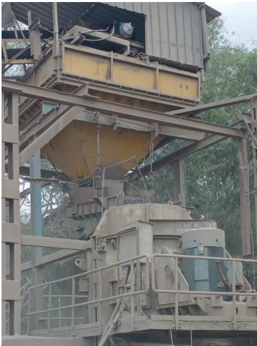
5a. Emissions at secondary crushing
