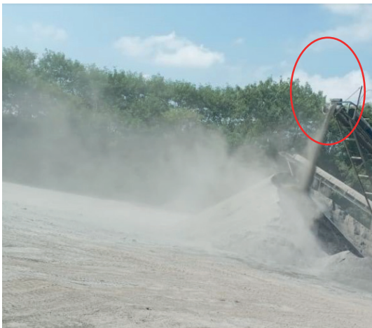
11a. Sprinkler not working near dust heap
