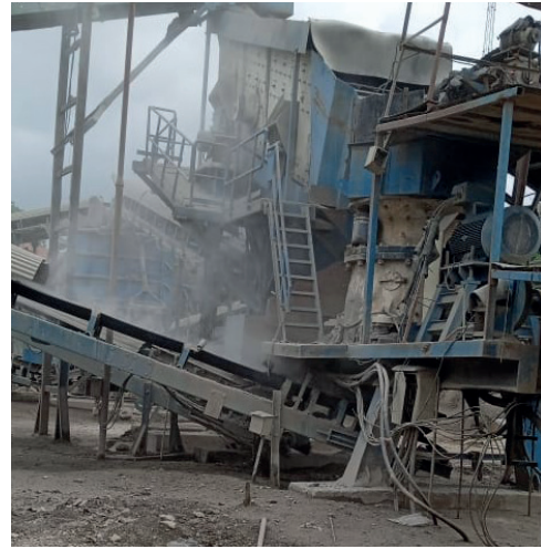
10b. Uncovered conveyor belts
