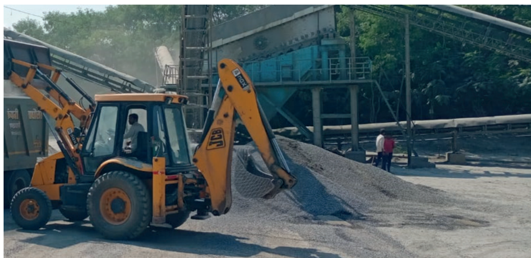
Image 7: Screening area covered with sheds, sprinklers not working
