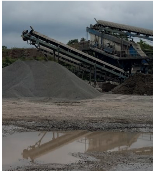
15b. Roads filled with water inside the crusher
