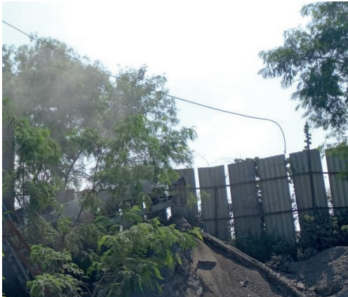
9a. Gaps between wind-breaking walls
