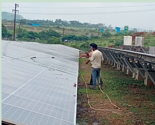
17a. Cleaning of solar panels
