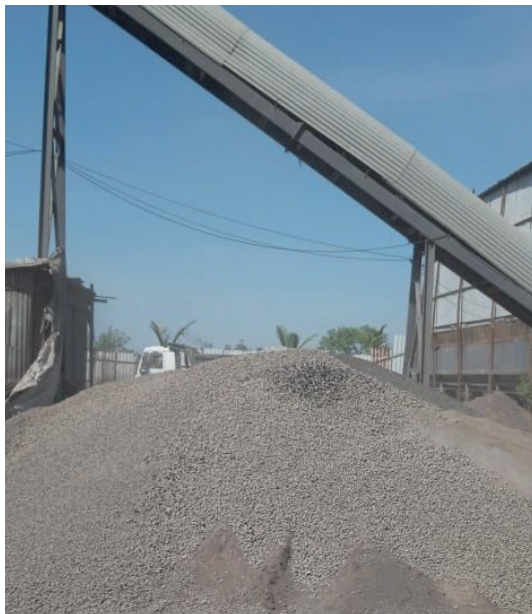
10c. Fully covered conveyor belts
