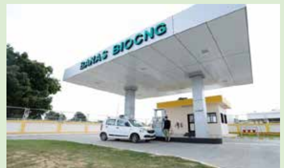
Bio-CNG dispensing unit ▲
