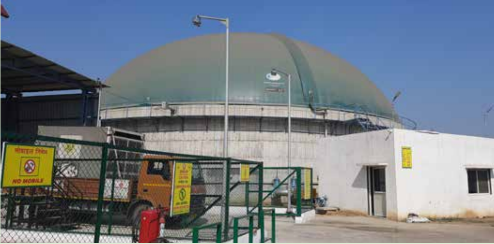
Biogas digester (Capacity: 4 TPD) ▲
