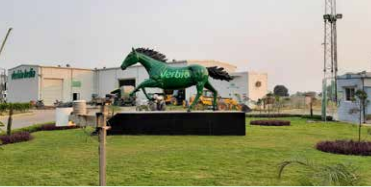
Verbio bio-CNG plant, (Weather monitoring system) ▲
