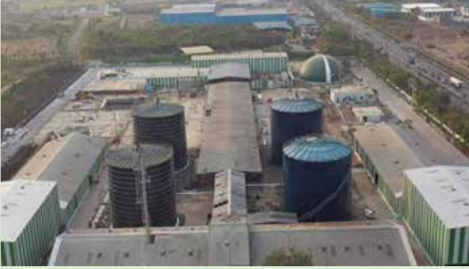
Overview of the Indore CBG plant ▲
