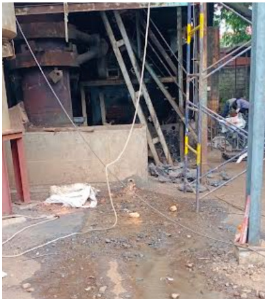
8a. Overflow from wet scrubber tank
