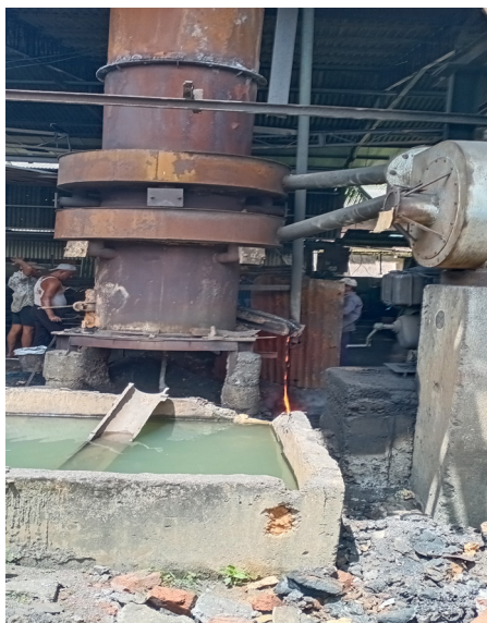
3a. DBC with wet scrubber
