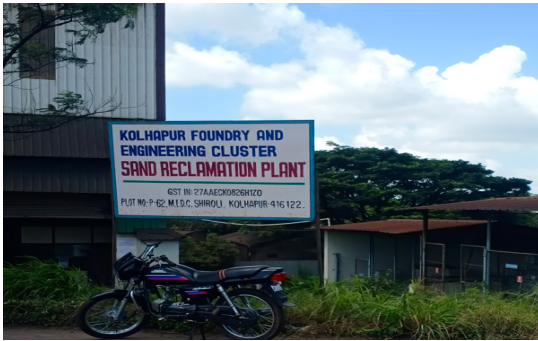
15a. Entrance of the sand reclamation unit
