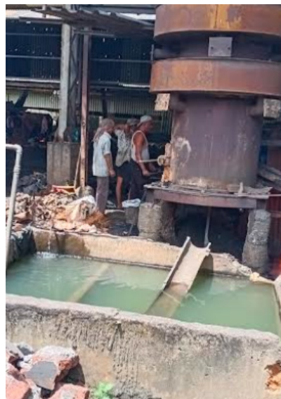
9b. Wet scrubber installed at a foundry
