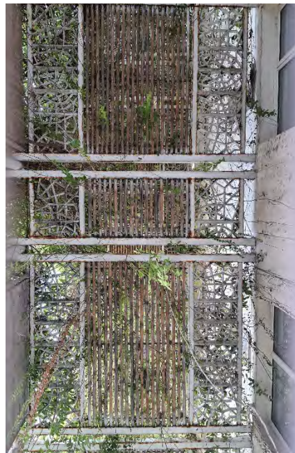
An external structure set a few feet away from the building envelope serves the dual purpose of working as a shading device while providing a medium for the plants to grow over, hence helping with the shade as well as enhancing microclimate through evapotranspiration for the western façade at IIPH Gandhinagar.
