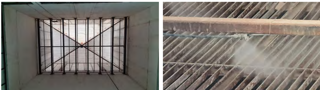
Fine water mist generated at the top of the tower by micro ionizers
