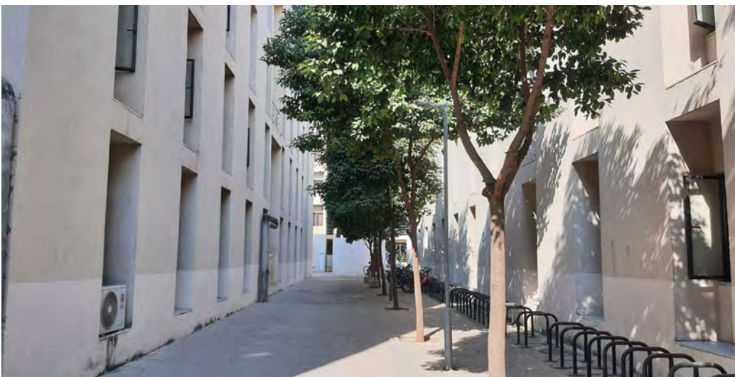
The proportions of the buildings and the distances between them have been kept as such that they allow for courtyard shading and mutual-building shading to take place.
