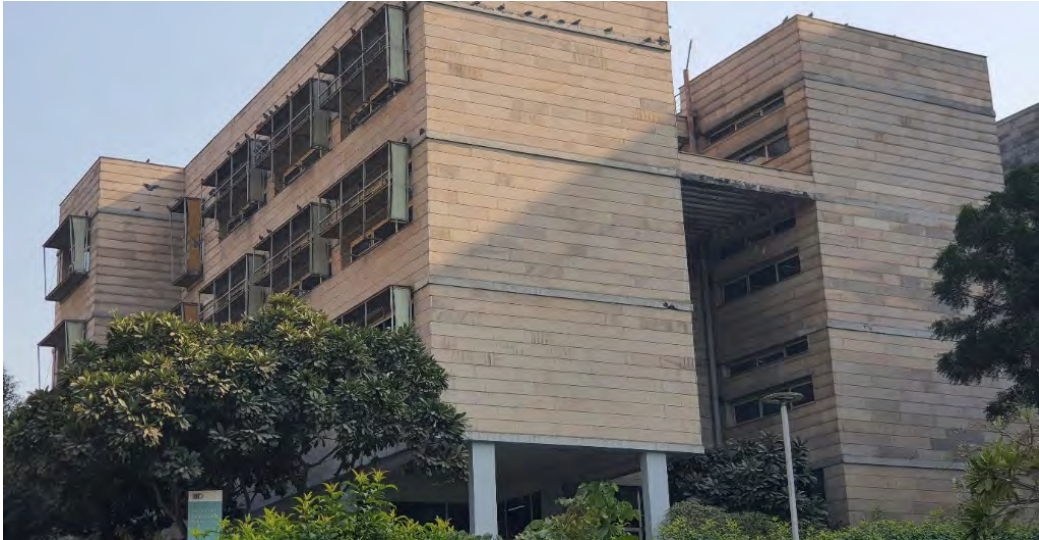
Elaborative shading devices for shading northern and southern facing windows while presenting a window-less façade towards East to minimize heat gains in IIIT, Delhi.
