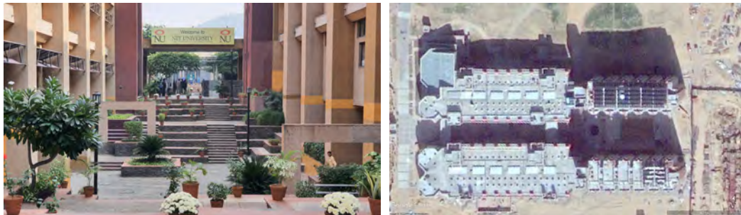
The distances between the buildings are kept narrow to ensure that the buildings mutually shade each other.
