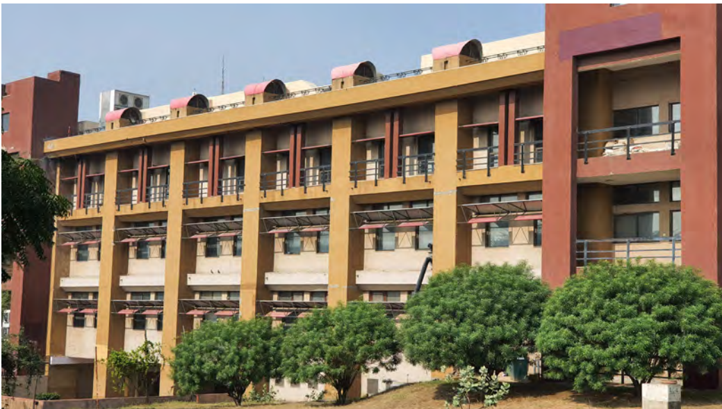
Warmed up air gets exhausted through the shafts and exits through cowls
