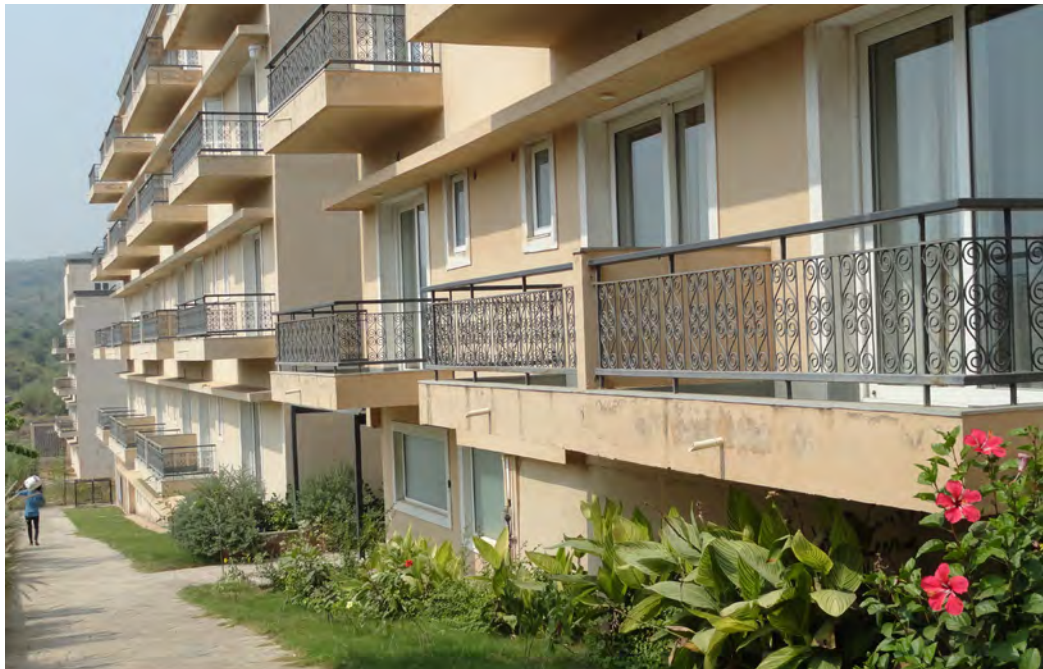
Projection factor of windows helps to shade during summer months and allows the winter sun to enter livable spaces.
