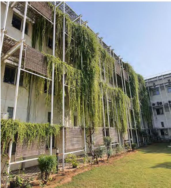
An external structure set a few feet away from the building envelope serves the dual purpose of working as a shading device while providing a medium for the plants to grow over, hence helping with the shade as well as enhancing microclimate through evapotranspiration for the western façade at IIPH Gandhinagar.
