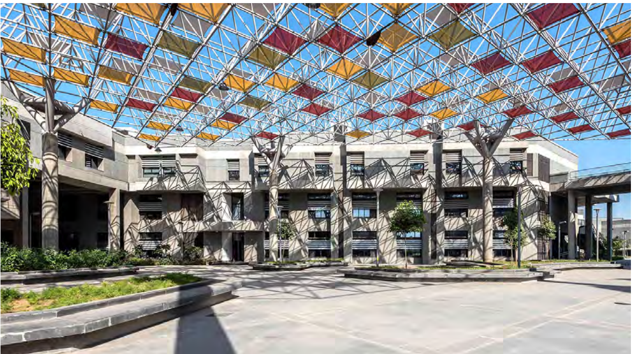
The central pergola acts as a shading device in the middle of the academic block
