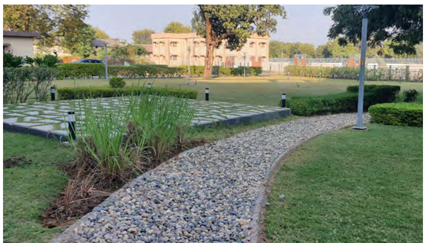
Pathways around the buildings have been kept permeable wherever possible so that less amount of heat gets absorbed by surfaces hence cutting down on the urban heat island effect.
