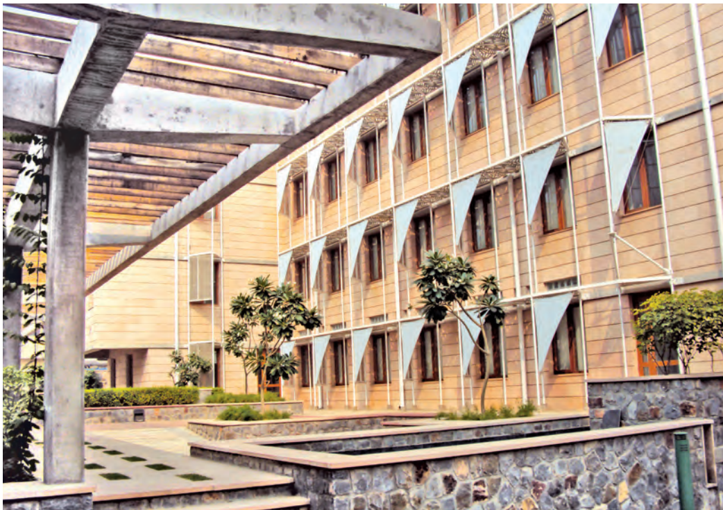
The Sehgal Foundation building in Gurugram has employed a radiant cooling system
