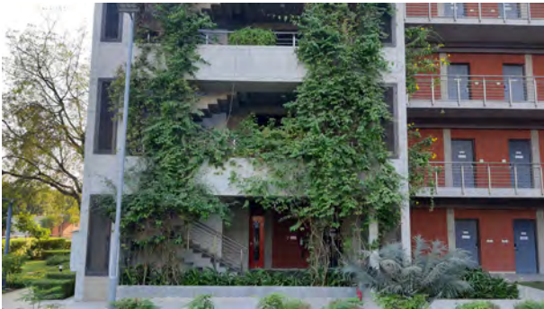
Vertical gardens have been used as a strategy that wraps around the building while shading and cooling the building facades and creating a cooler microclimate.
