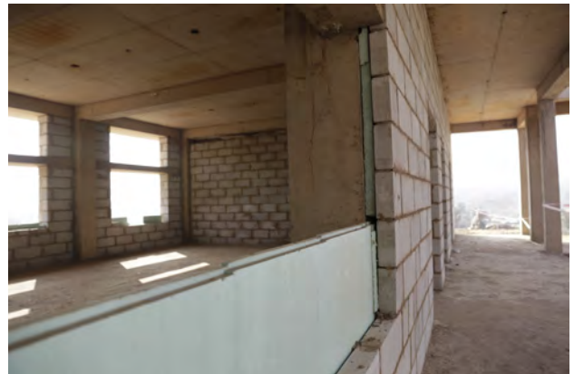
350mm wall with combination of AAC blocks and XPS insulation
