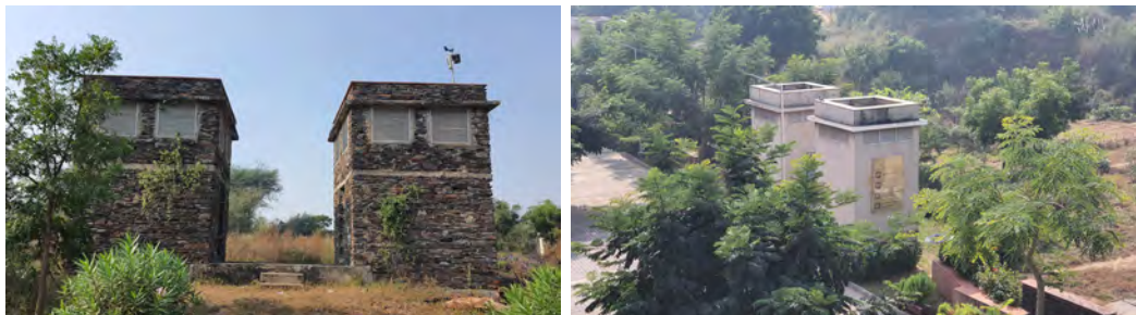
Wind intake towers
