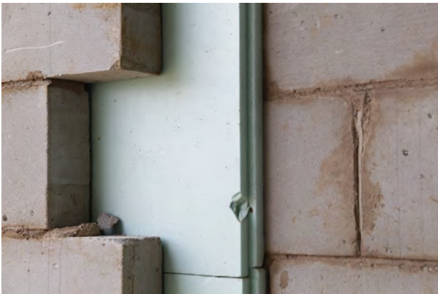
350mm wall with combination of AAC blocks and XPS insulation
