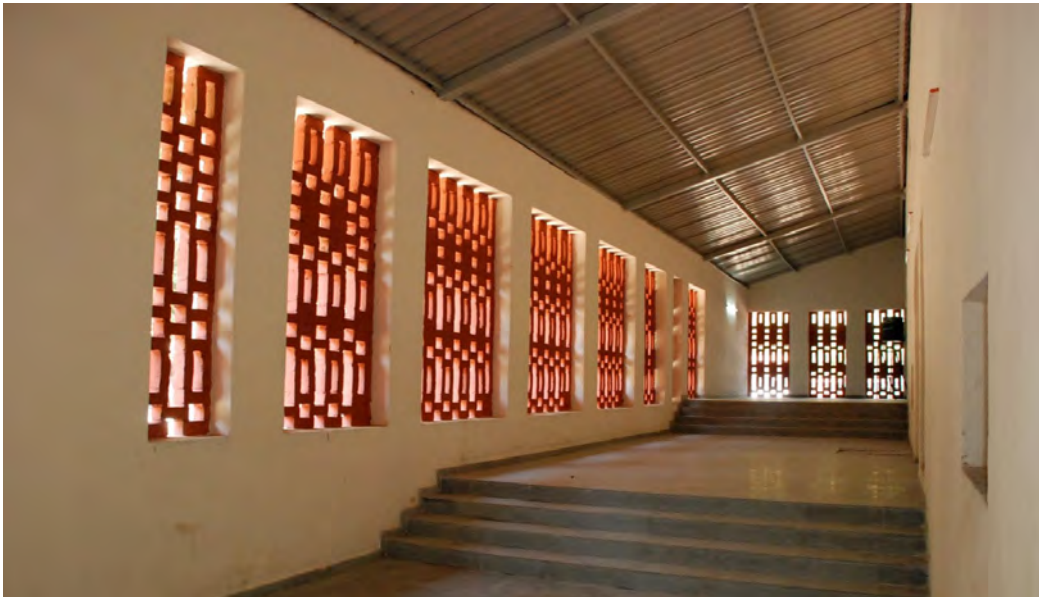
A double skin facade protects the interior spaces by adding a buffer zone
