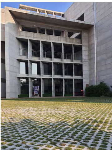
Pathways around the buildings have been kept permeable wherever possible so that less amount of heat gets absorbed by surfaces hence cutting down on the urban heat island effect.
