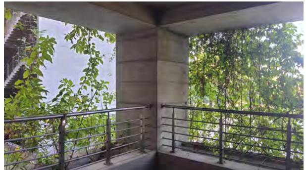
Vertical gardens have been used as a strategy that wraps around the building while shading and cooling the building facades and creating a cooler microclimate.
