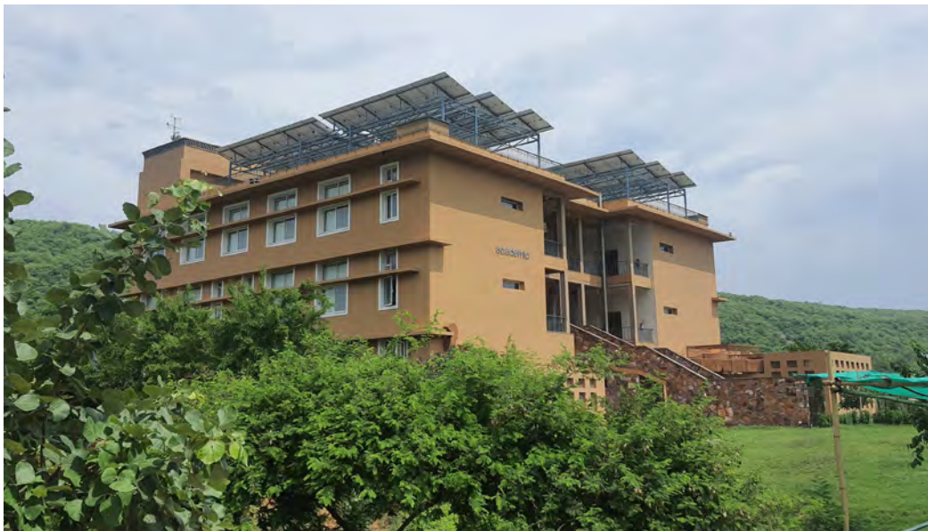
The western façade receives the brunt of the harsh summer sun; the classrooms are shielded from this by utilizing washrooms as buffer zones in academic block.
