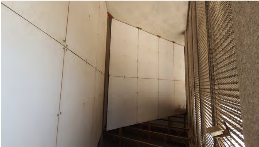
Air gets filtered at the top of the tower
