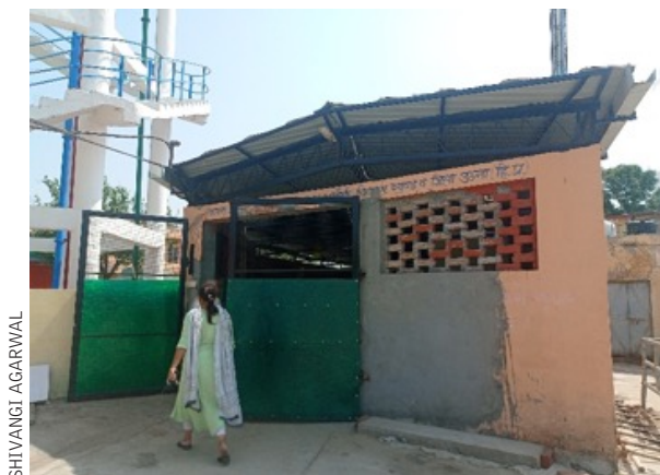
Photograph 15: Waste segregation shed
