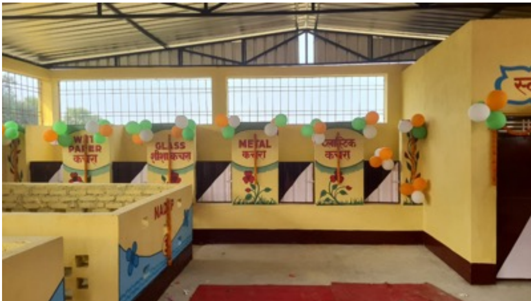
Photograph 8: Waste segregation shed at Nawan gram panchayat.
