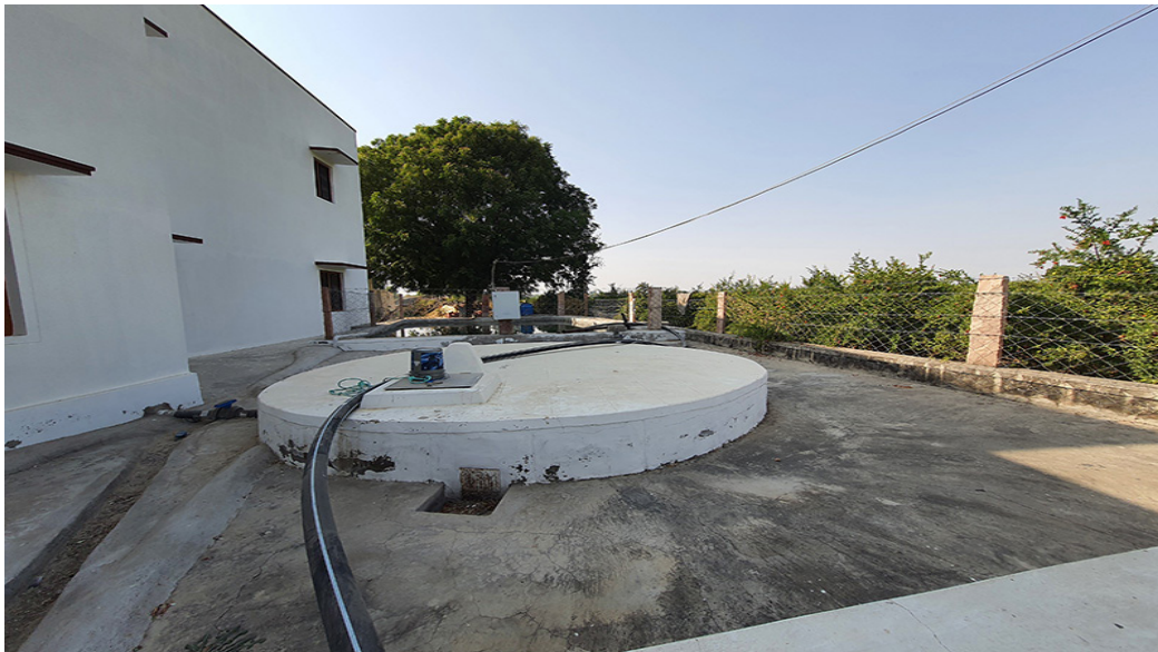
Rooftop rainwater-harvesting system connected to a tanka, Budiwada village, Barmer district, Rajasthan
