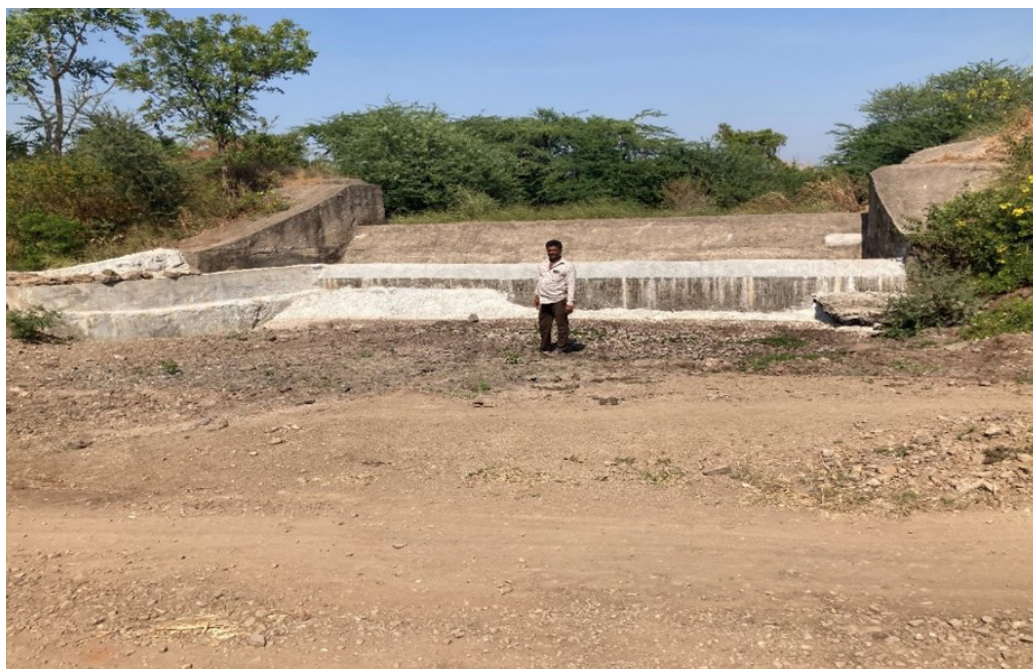
The Cement Nala Bund constructed by the community in Mota Munjiyasir village in Bagatsara tehsil, Amreli district
