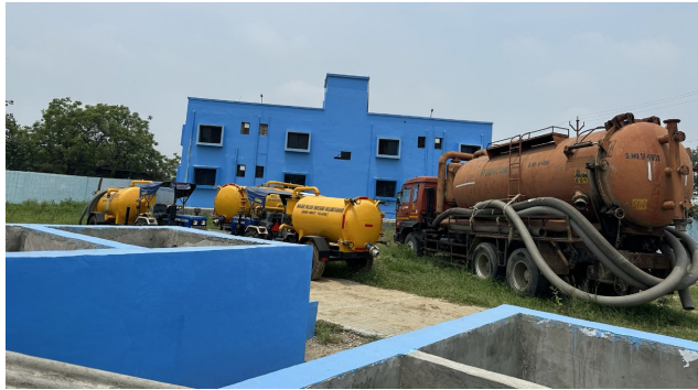
Co-treatment plant in Bulandshahr
