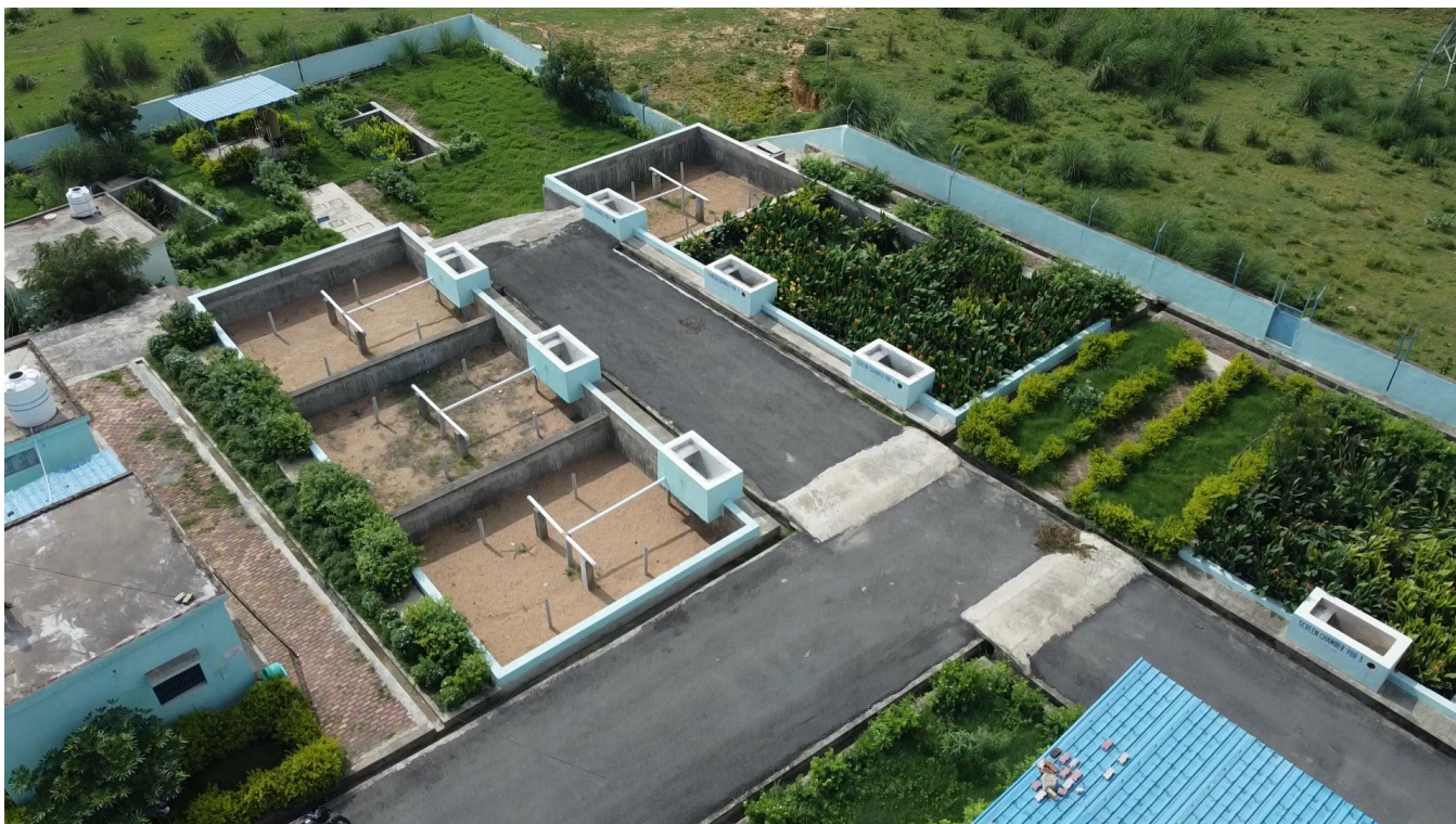
Faecal sludge treatment plant (FSTP) at Chunar
