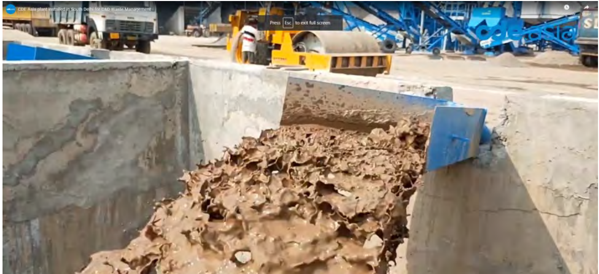
Sludge being poured into the siltation tank
