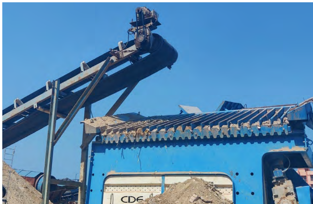
Secondary crushing stage which prepares the waste feed for wet processing
