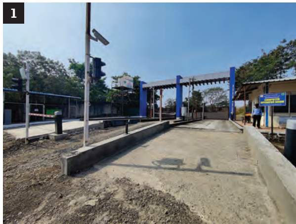
C&D waste recycling plant at Moshi
