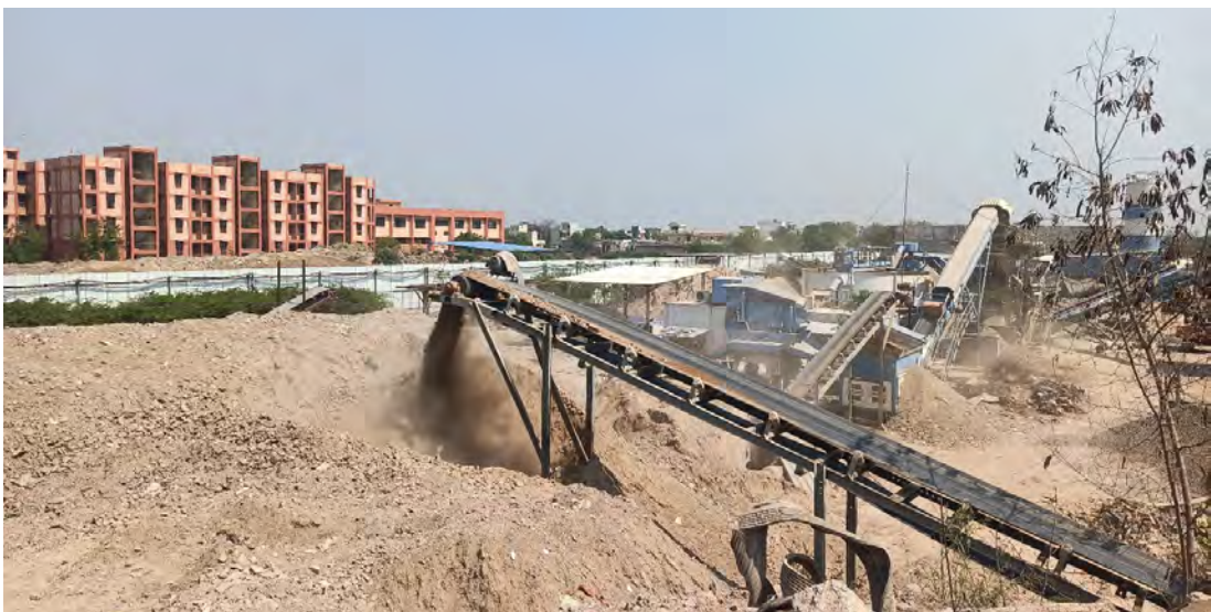
Conveyor belt carries pieces smaller than 60 mm after preliminary crushing
