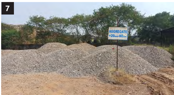
7. Processed aggregate stored on site; 8. Different types of processed re-usable aggregates
