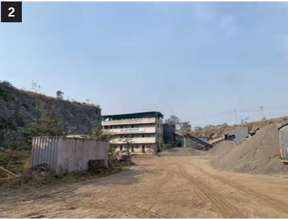
2. Untarred/Unpaved roads within the C&D plant at Wagholi
