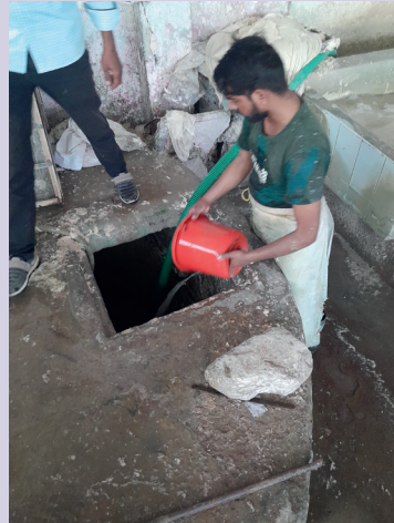
Pulp storage tank
