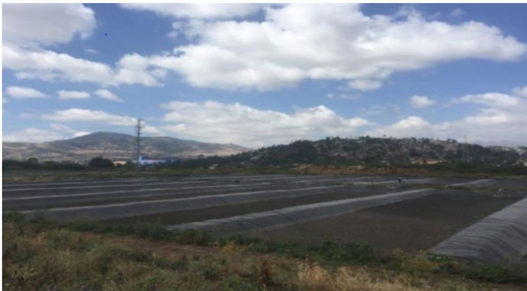
Drying bed for faecal sludge in Kality
