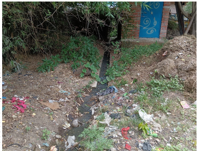
Grey water flows through improper drains in Sidhauna village, Amanwa block.
