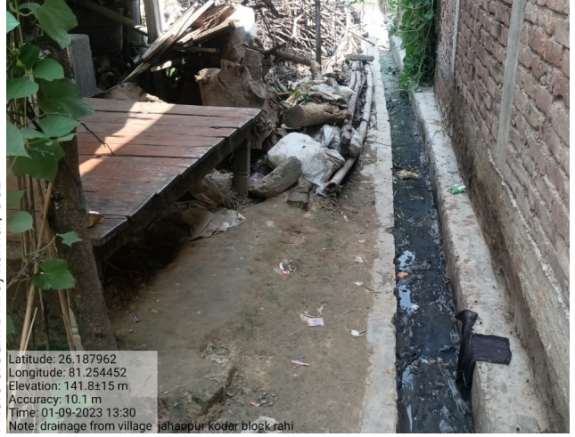
Existing drains are silted or lack maintenance in Jahanpur Kodar village, Rahi block
