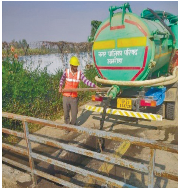
Sludge being received at the Amroha plant
