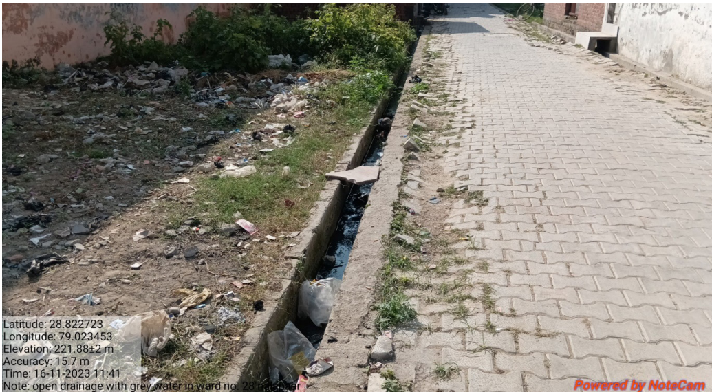
The narrow undersized drains in the Nalapaar area (ward number 28) of Rampur are choked with plastic, and greywater from households flows unabated into the drains. Spilling of wastewater is a common issue in the area after the rains.
