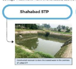
After the treatment from the STP, the treated water is stored in a reservoir. This water is distributed to farmers in Chhapra village through underground pipelines that stretch for a distance of 10,950 meters.
