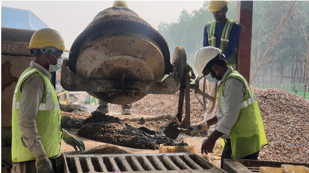
Image 38: Concrete mixture unit
