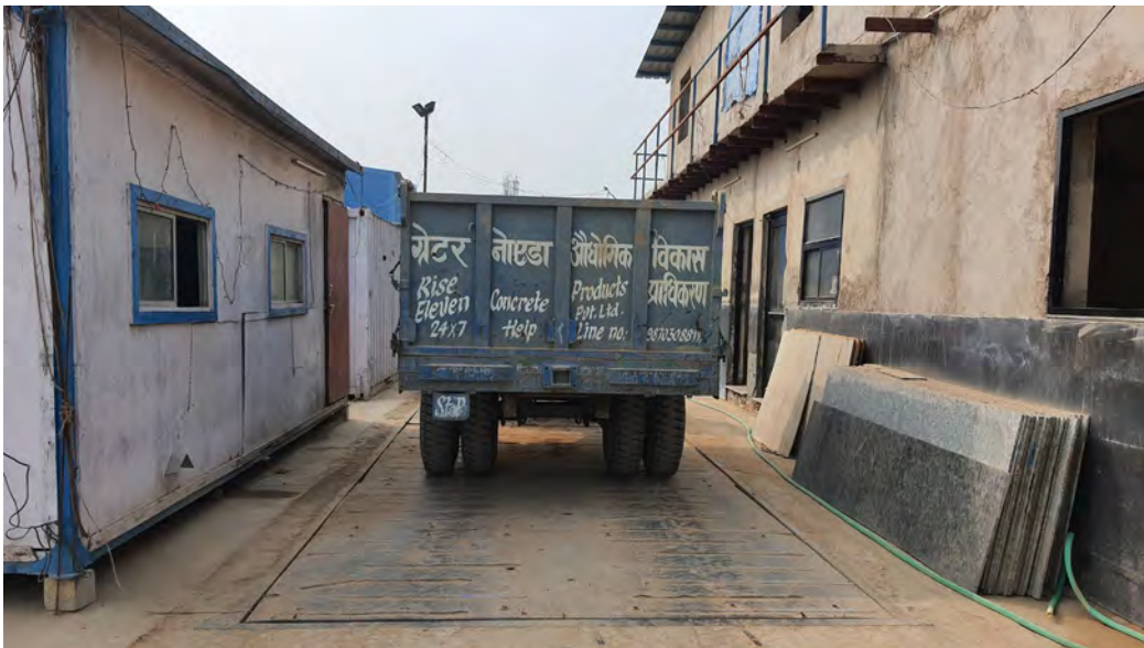
Image 20: Weighing bridge at Greater Noda C&D recycling plant
