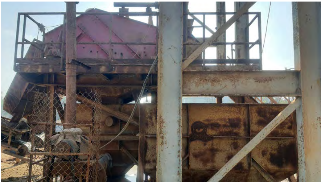
Image 32: Hydrocyclone at Gurugram plant
