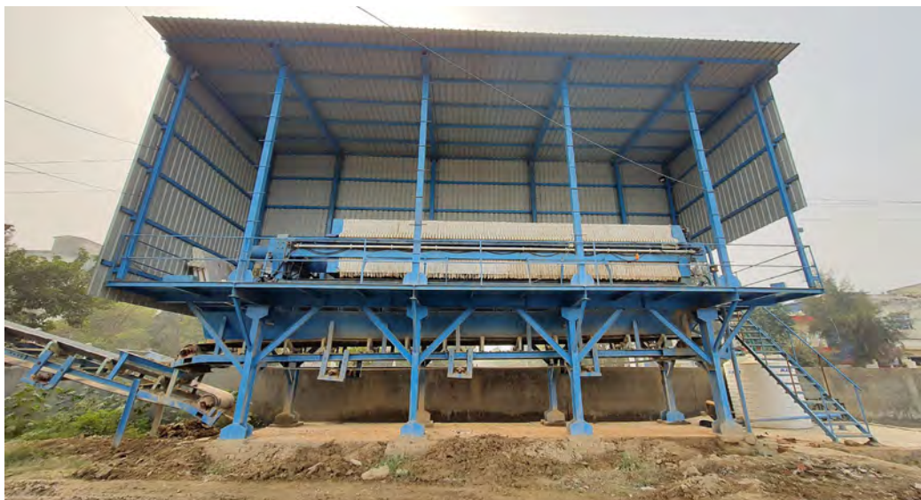
Image 34: Filter press at Greater Noida plant
