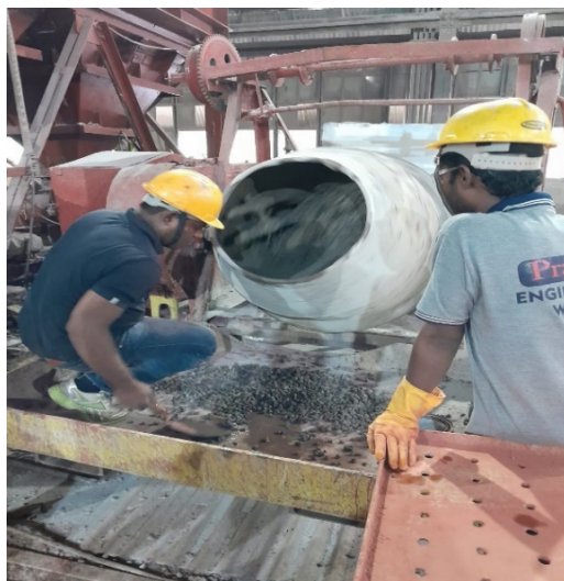
Proportioning and mixing
