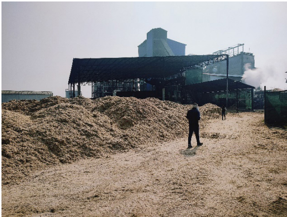
Bagasse storage yard
