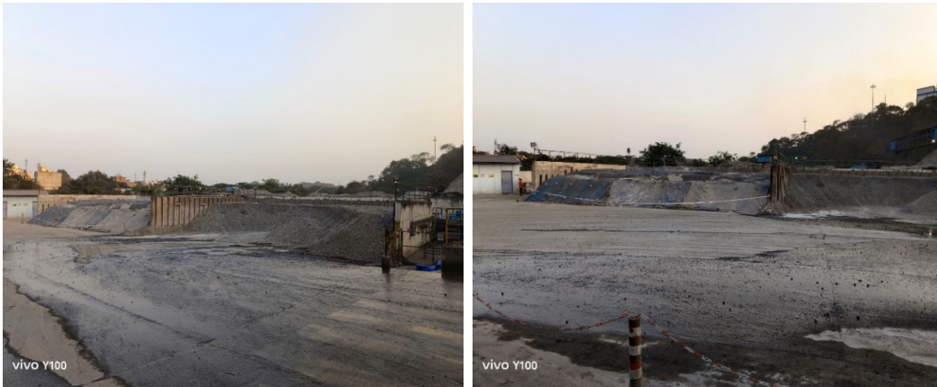
Steam ageing plant at Tata Steel Jamshedpur
