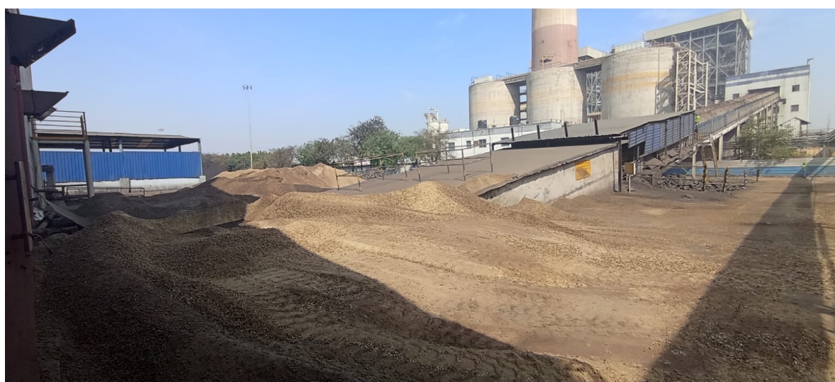
Biomass feeding point at Jhajjar Power Limited
