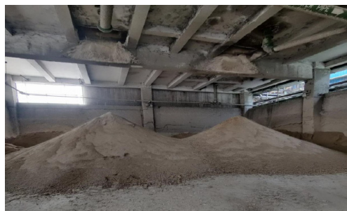
FGD gypsum storage in Jhajjar Power Station
