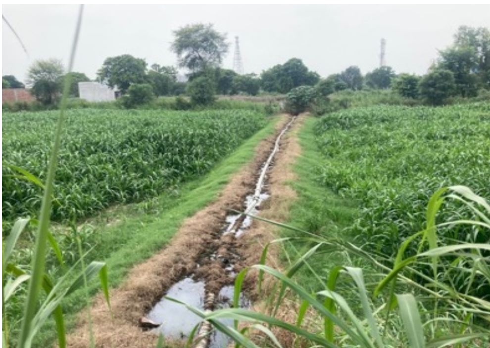
Pipeline network laid by farmers in Dhandupura village, Agra taking treated water from access point to their field.
