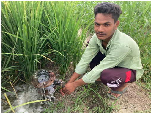
Farmer accessing treated water from hydrant installed in the field for agriculture in Baraichpur village, Kurukshetra District, Haryana
