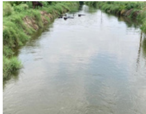
Canal which carries the treated water from Jajmau, STP
