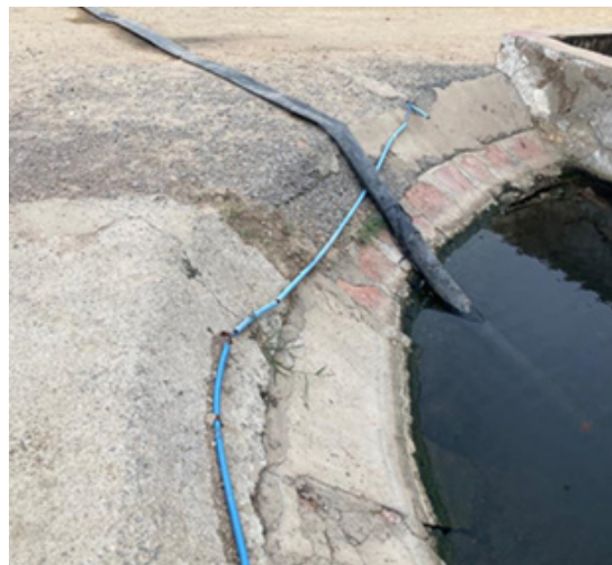
Pipeline laid by farmer in Nagla vihari village to extract water from oxidation pond in Peelakhar STP
