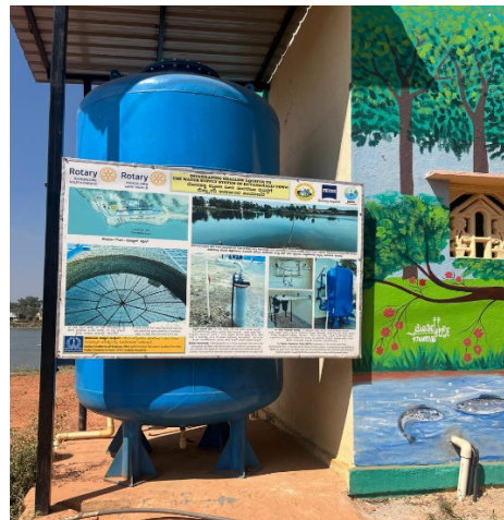
Water treatment plant near Sihineeru lake to treat the open well and borewell water before supply
