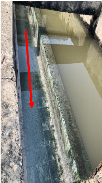
Channel for treated effluent from where the water flows in pipeline for disposal in Anasagar lake
