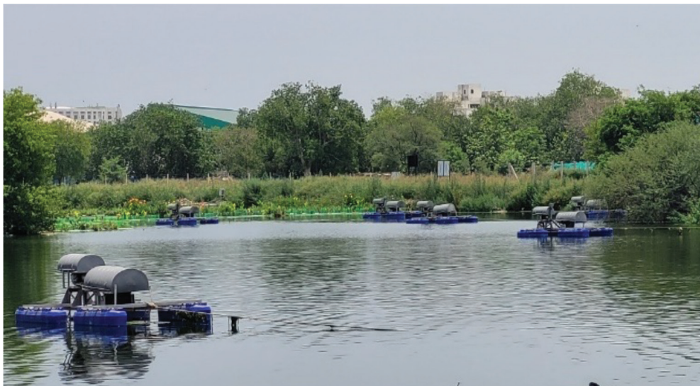
Artificial lake in the premises of Pappankalan Sewage Treatment Plant in Dwarka, Delhi receiving treated water for lake recharge.
