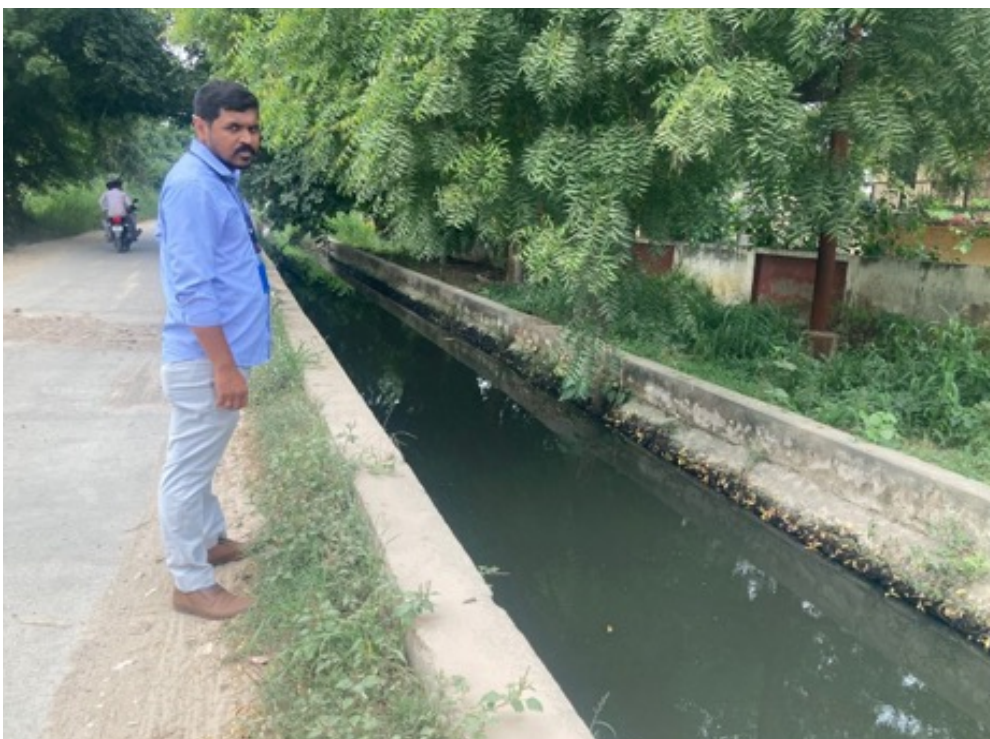
The open canal adjacent to the Dhandupra STP where treated water is discharged to be used by farmers for agriculture.
