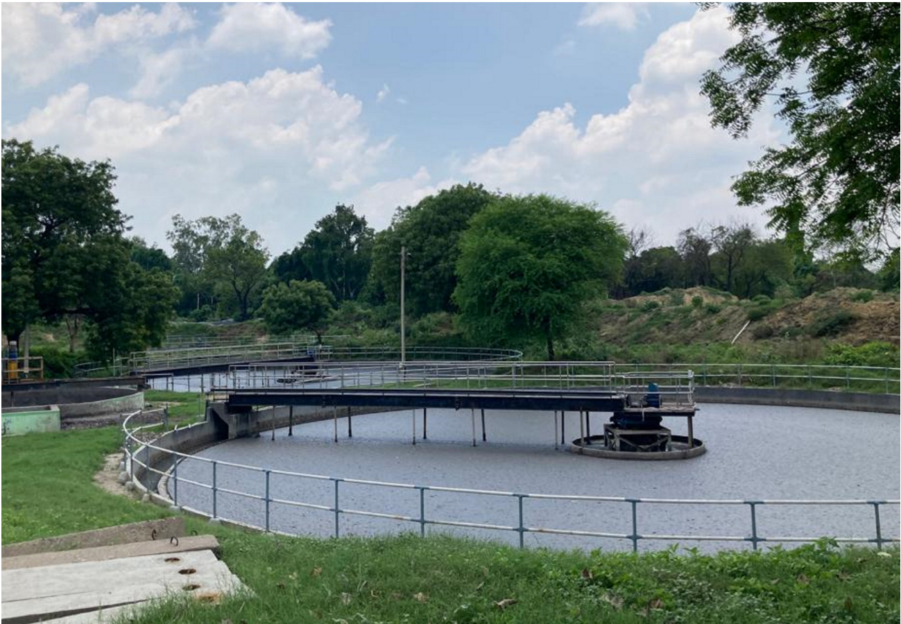
Jajmau STP in Kanpur. The treated wastewater from this STP is channelled into a nearby escape canal from where the water is tapped for agriculture by the farmers using gravitational force.
