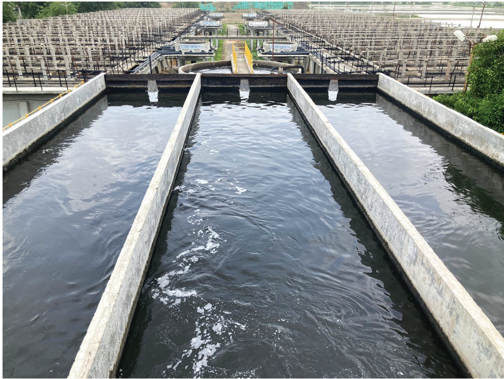
Dhandupura STP, located in Agra, was commissioned in 2001. It has a total treatment capacity of 78 MLD. The treated wastewater from this STP is discharged into a nearby canal from where the farmers tap the water for agricultural purposes.
