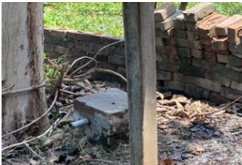
Opening in field through underground pipeline from where the treated water is extracted by farmers in Bhagwanpur, Varanasi
