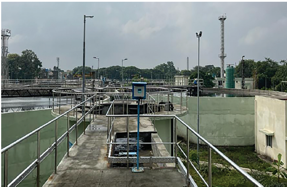
Nasapakkam Secondary Treatment Plant; treated water from this plant feeds into the tertiary treatment plant
