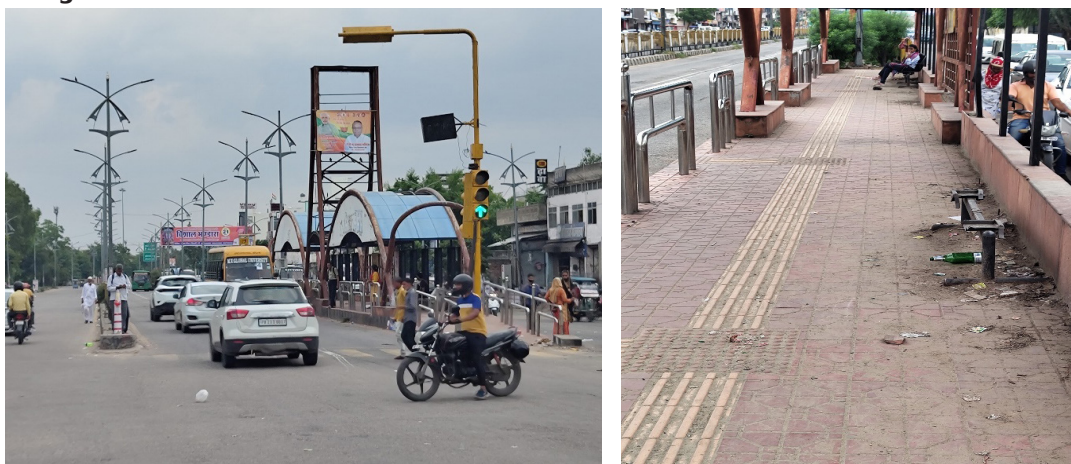
Image 3: Poor condition of BRT corridor
