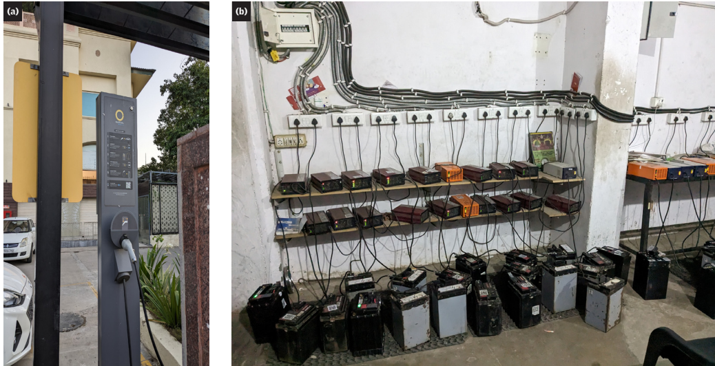
Figure 3: a) Sunfuel Electric DC charger, b) Dockless battery swapping centre for e-rickshaws
