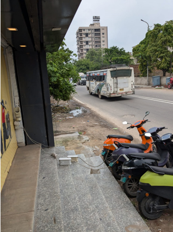
Figure 4: AC socket charging of Ola E-2W
