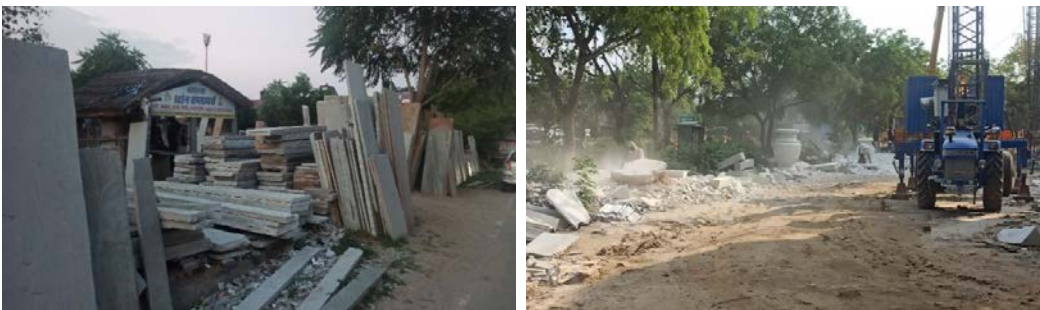
Stone slab material store (left); Fugitive dust formation during stone work at a site near Jaipur's airport (right)
