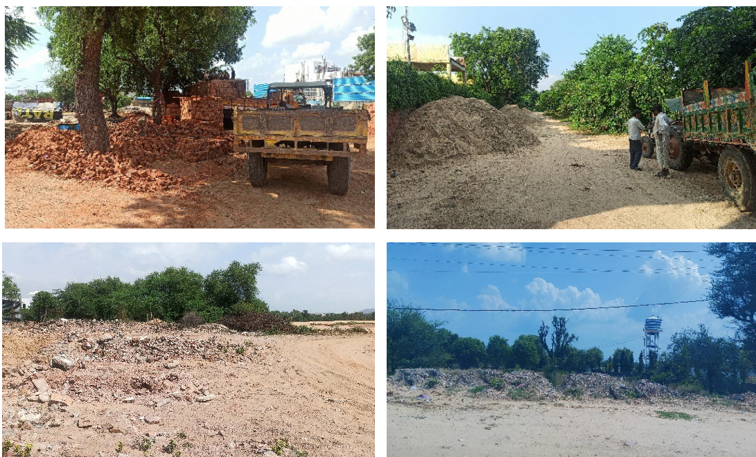
Material mandi without any dust control measures (left); illegal C&D waste dumping sites (right)
