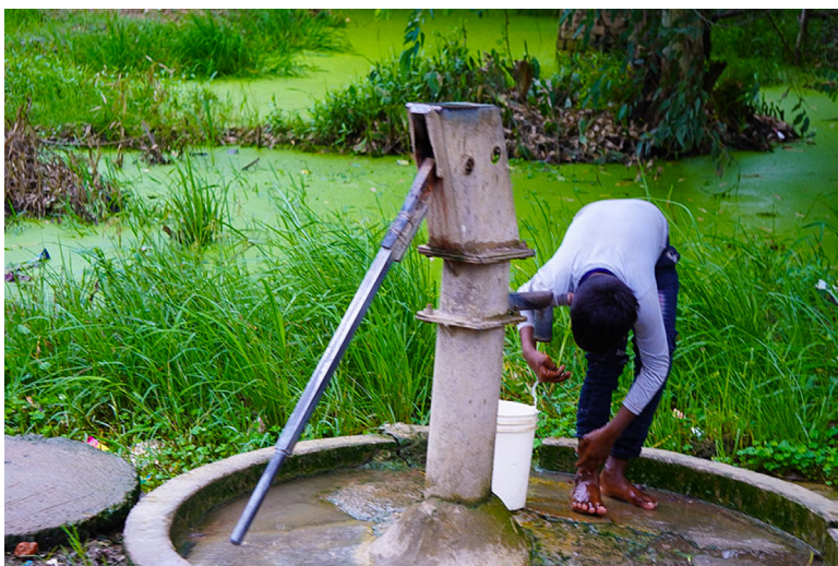
Grey water from handpumps directly discharging into nearby depressions and ponds due to faulty design of community soakpits.
