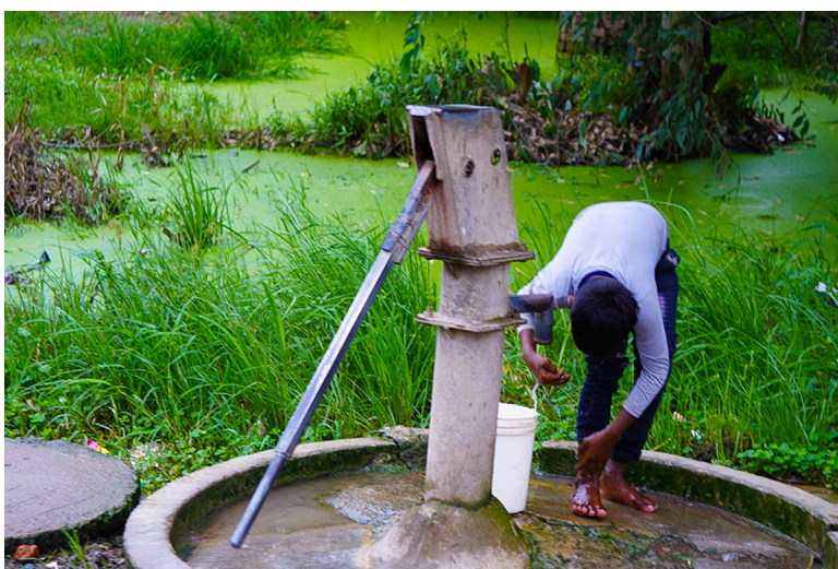
Grey water from handpumps directly discharging into nearby depressions and ponds due to faulty design of community soak pits.
