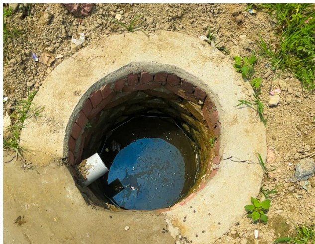
Grey water is not managed properly, and the stagnant water breeds mosquitoes in Bhandpura in Chamrauwa block.
