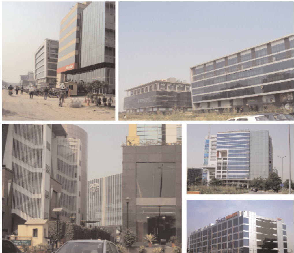
Fig 28: Snapshot of Buildings in Central Business District in Jasola
