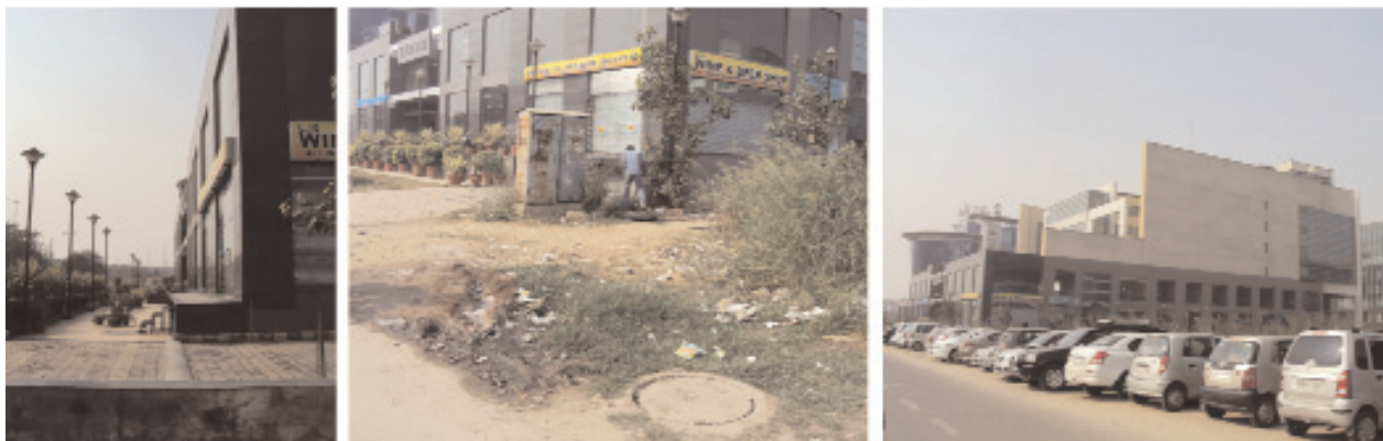
Fig 29: Parking, Green belt and Drainage issues around TDI Centre
